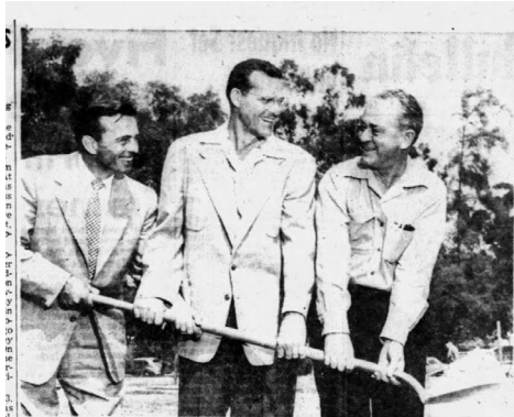
GROUNDBREAKING —Picking up a shovelful of Chino earth to break ground for the community's new civic center are architect Stanley Clark Meston, Mayor Howard Comstock and Contractor J. B. Campbell. The center is to be built in the city park. Ground for it was broken officially on Friday afternoon (P-B photo)
