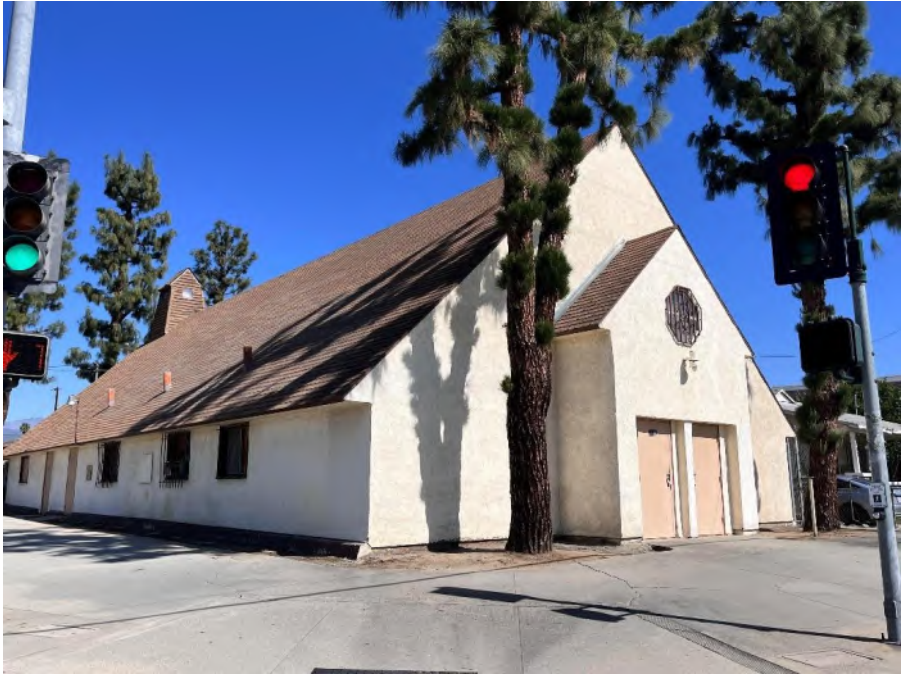
Exhibit 47. Sacred Heart Church, 1095 West Grand Ave, constructed 1935
