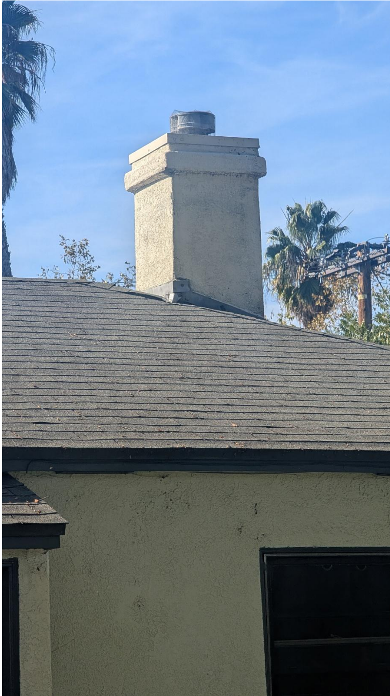
Project description: Chimney (stucco) on northerly side of dwelling.
