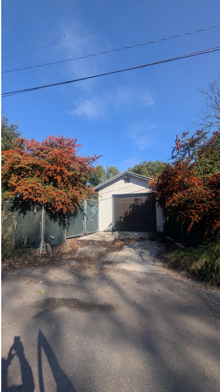
Project description: Subject site, rear yard, garage structure.
