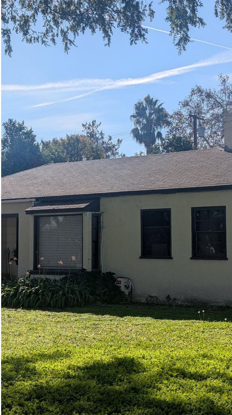
Project description: Subject site, front façade – windows.
