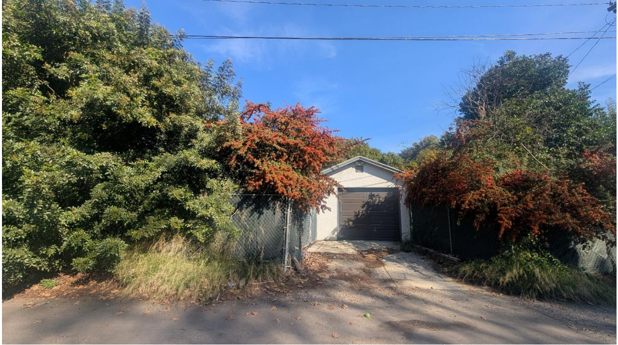
Project description: Subject site, rear yard, garage structure.
