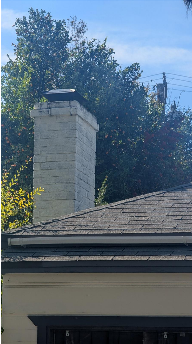
Project description: Chimney (brick material) on southerly side of dwelling.
