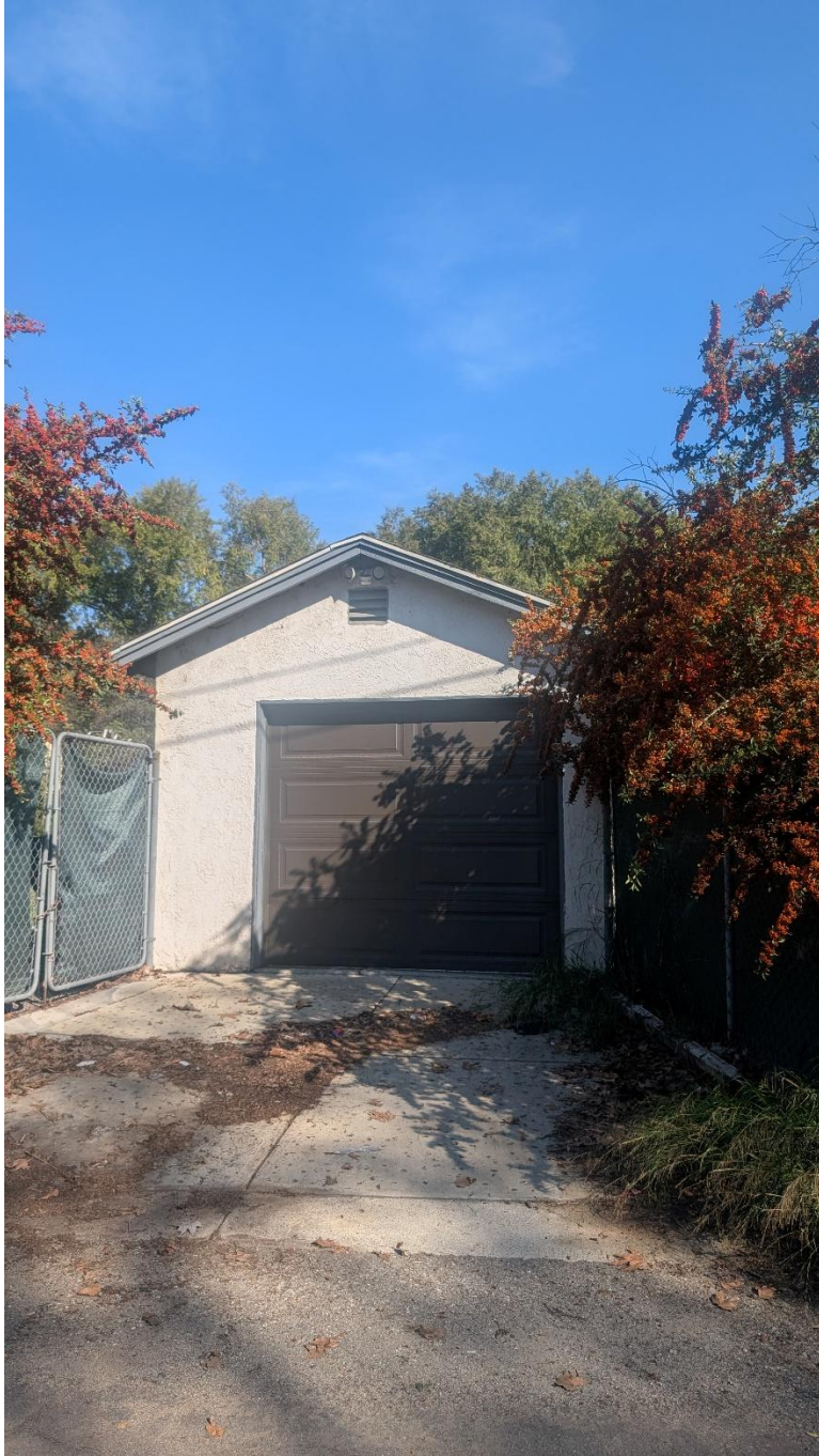
Project description: Subject site, rear yard, garage structure.
