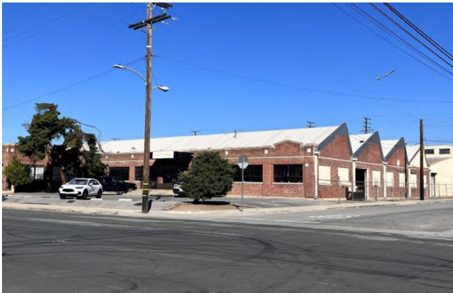
Exhibit 46. Example of Brick Industrial/Agricultural Building, Brogdex Fruit Building, 1441 West Second Street
