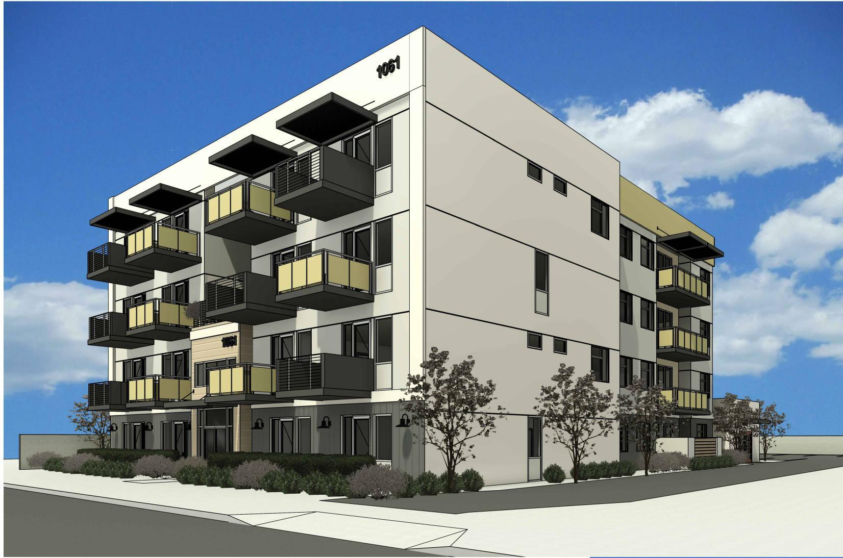
VIEW LOOKING NORTH-WEST
