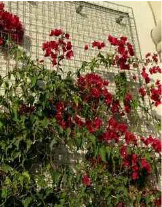
VINE GREEN SCREEN SYSTEM ANCHORED TO WALL
