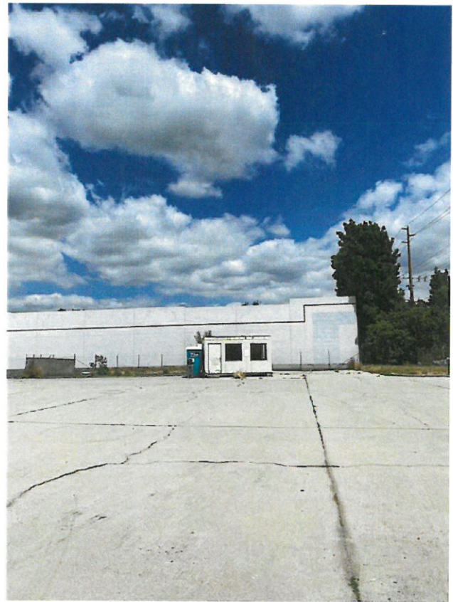
8. Eastern perimeter of the site looking at the adjacent warehouse.
