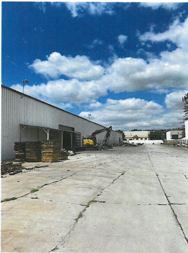
7. Eastern side of the existing building.
