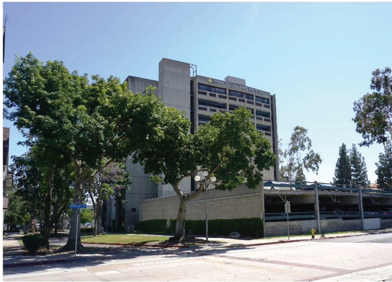
Speidel Building, 2022. HRG.
