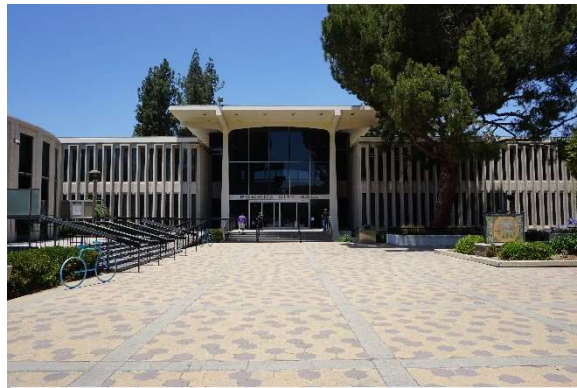
Pomona City Hall, 505 S. Garey Avenue (1969; Pomona Civic Center Historic District).
