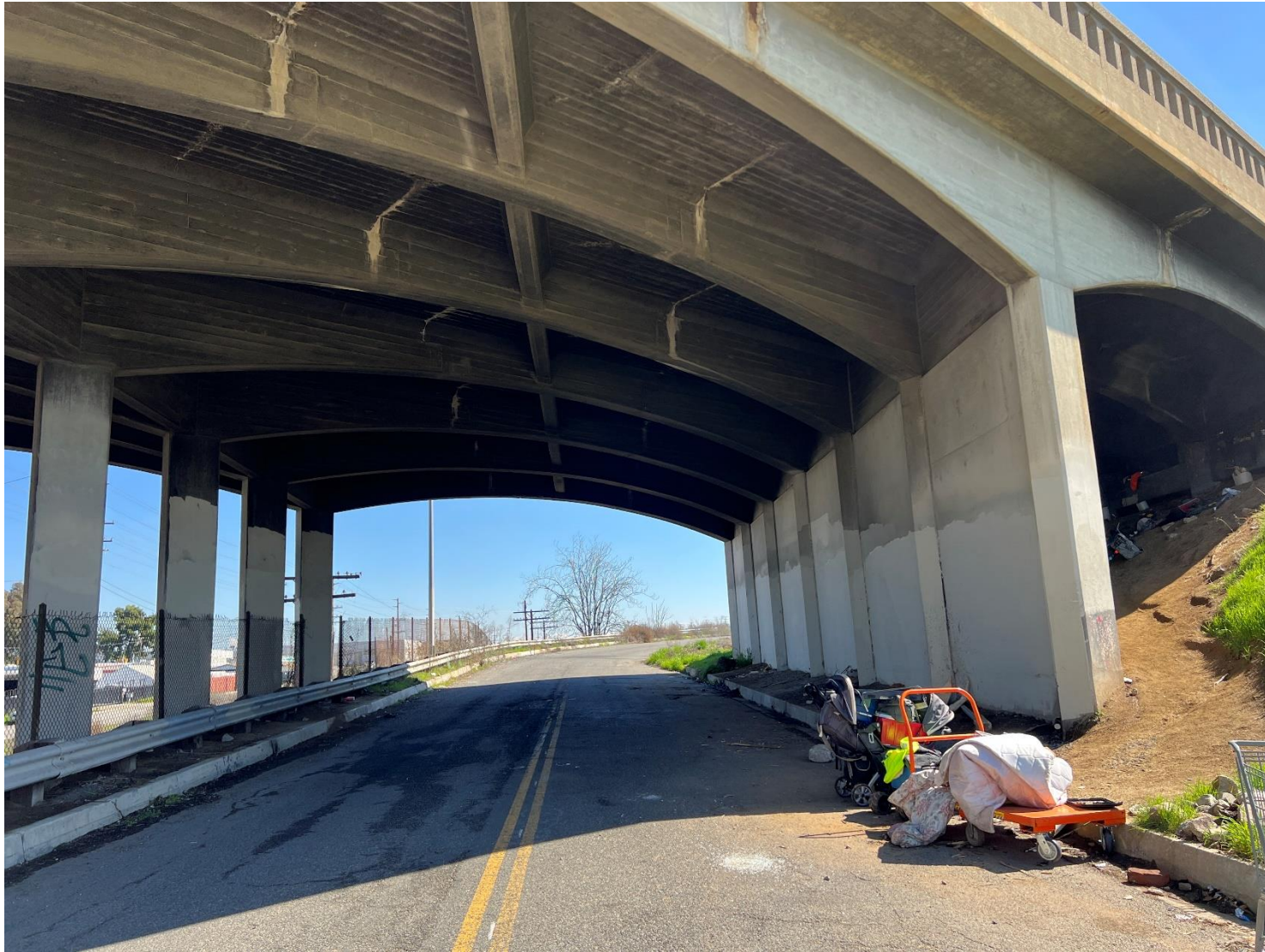
Figure 1 February 22, 2024 Pomona Blvd Right-of-Way with the 71 FWY Above
