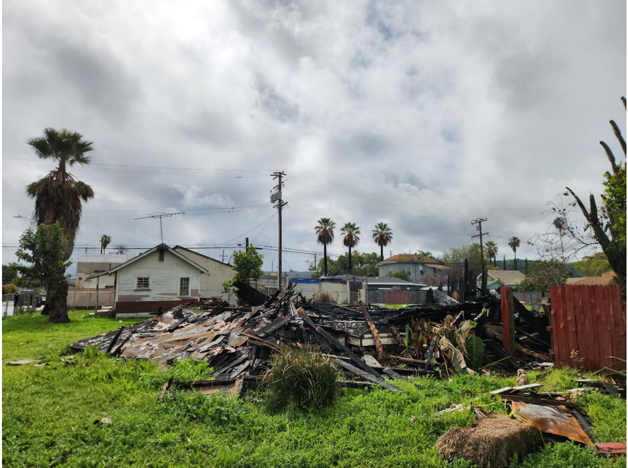
Adjacent property to north (115 S. Myrtle Avenue). Destroyed due to fire late 2025
