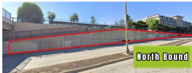
These walls total approximately 8,278 SQFT.
