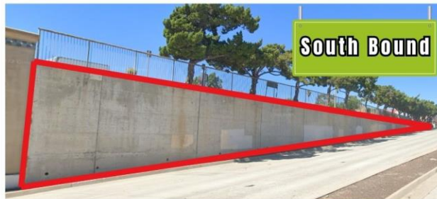
Area 1: Roadway Murals
