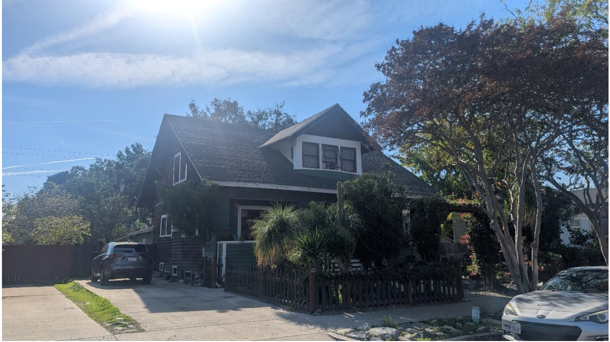
Project description: Front façade and side yard.
