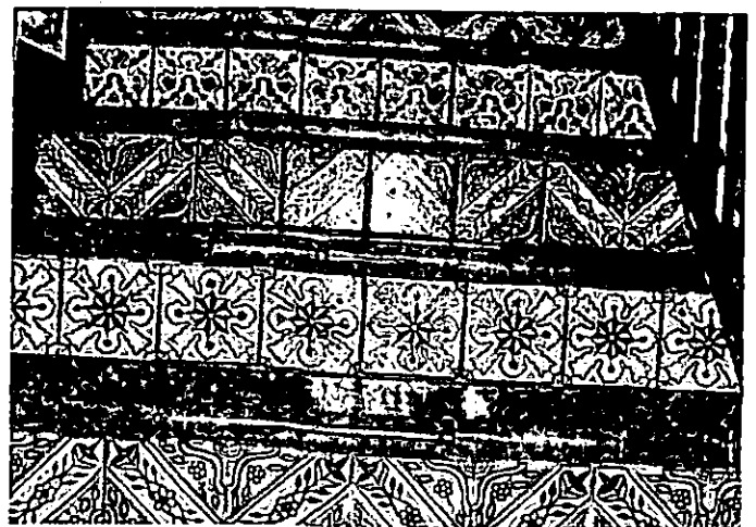
Stair Risers. Entry Reception Room. Tile. 6/2011.
