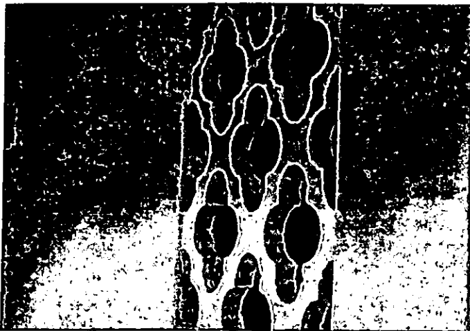
Window Grillework. Various locations. Masonry. 6/2011.
