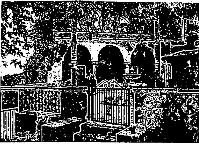
1300 Los Robles Place. Courtyard.
