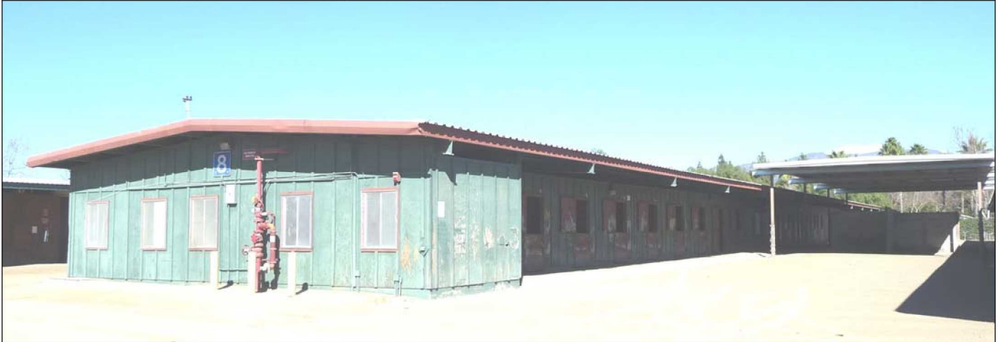
HRS #8 and metal canopy, view to the north (1/21/2011)
