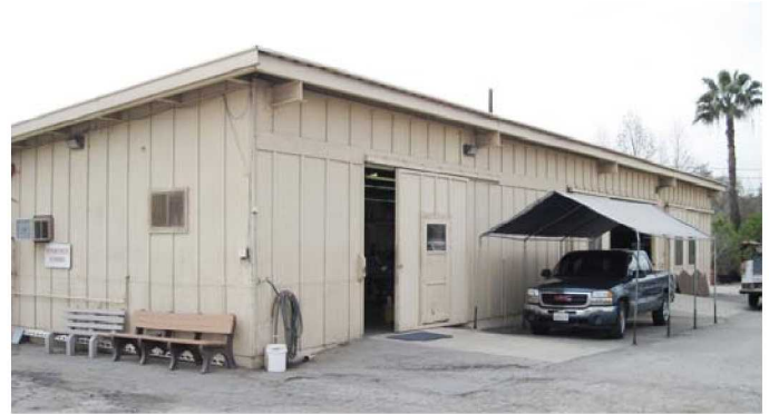
Building 5, view to the south (3/2/11)
