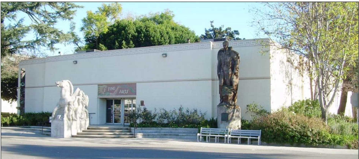
Figure 20: Millard Sheets Building, north elevation, view to the southeast (1/21/11).
