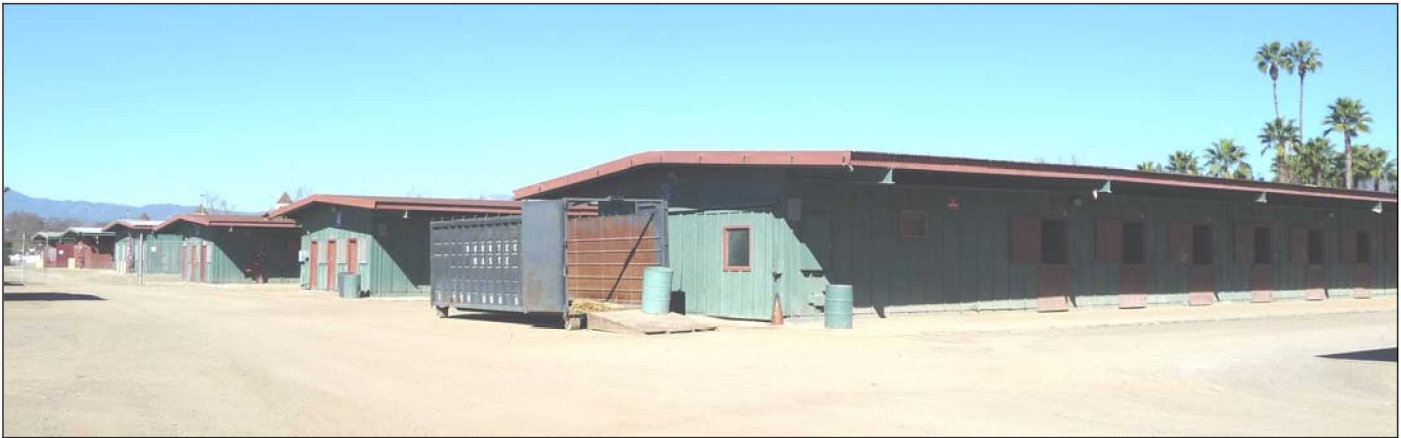
Overview of northern row of stables (HRS 1-12A), view to the northwest (1/21/2011)
