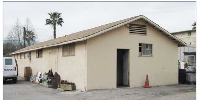
Building 6, view to the southwest (3/2/11).
