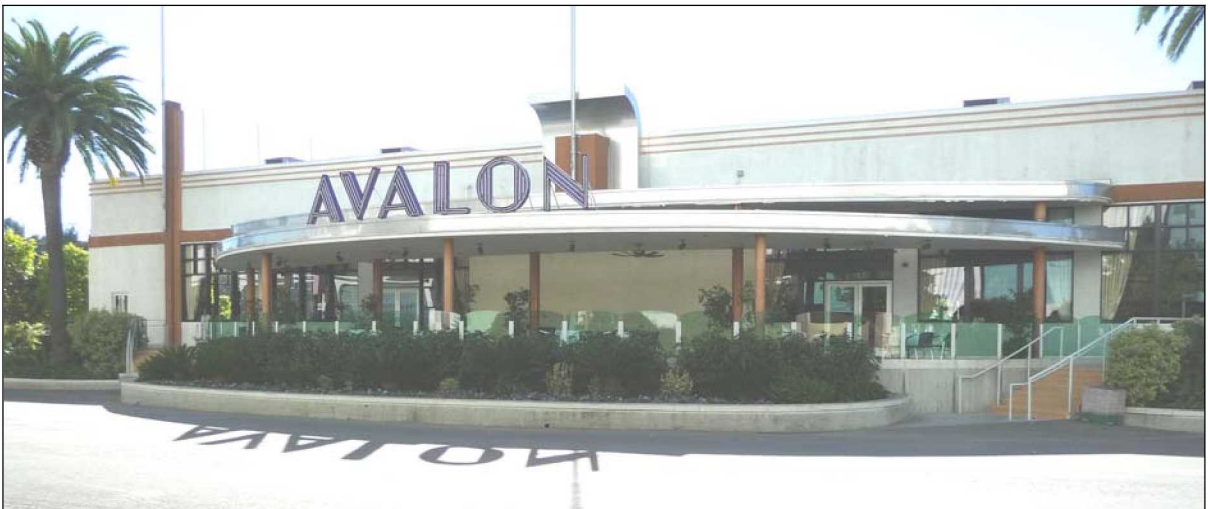
Figure 27: Avalon, east elevation with modern canopy/patio cover (1/21/11).
