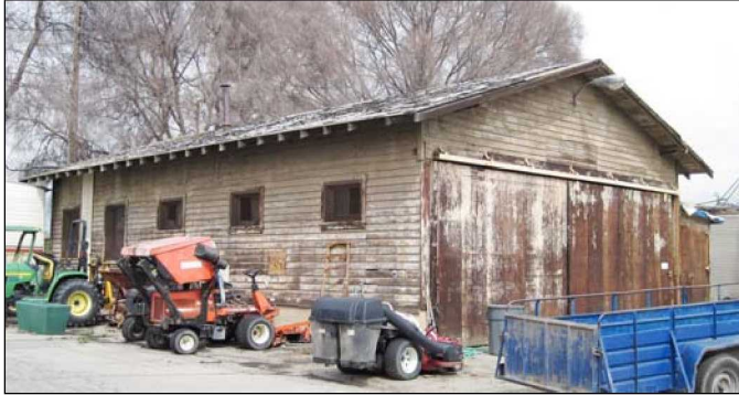
Building 8, view to the northeast (3/2/11).
