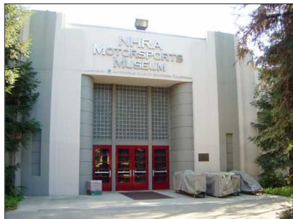
Figure 32: NHRA Motorsports Museum, north elevation entrance (1/21/11).
