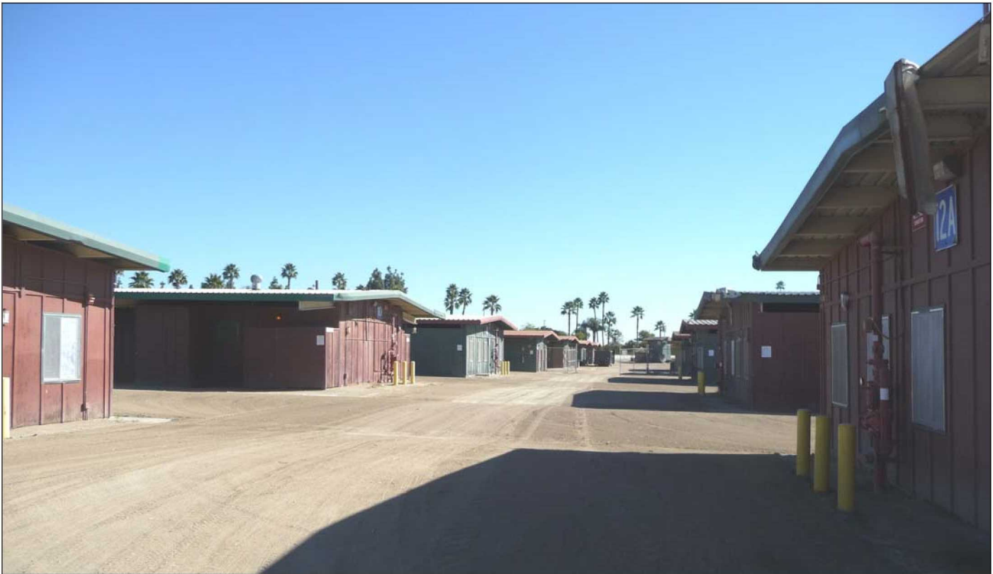
Central corridor between Horse Racing Stables 1-12A, view to the east (1/21/2011)
