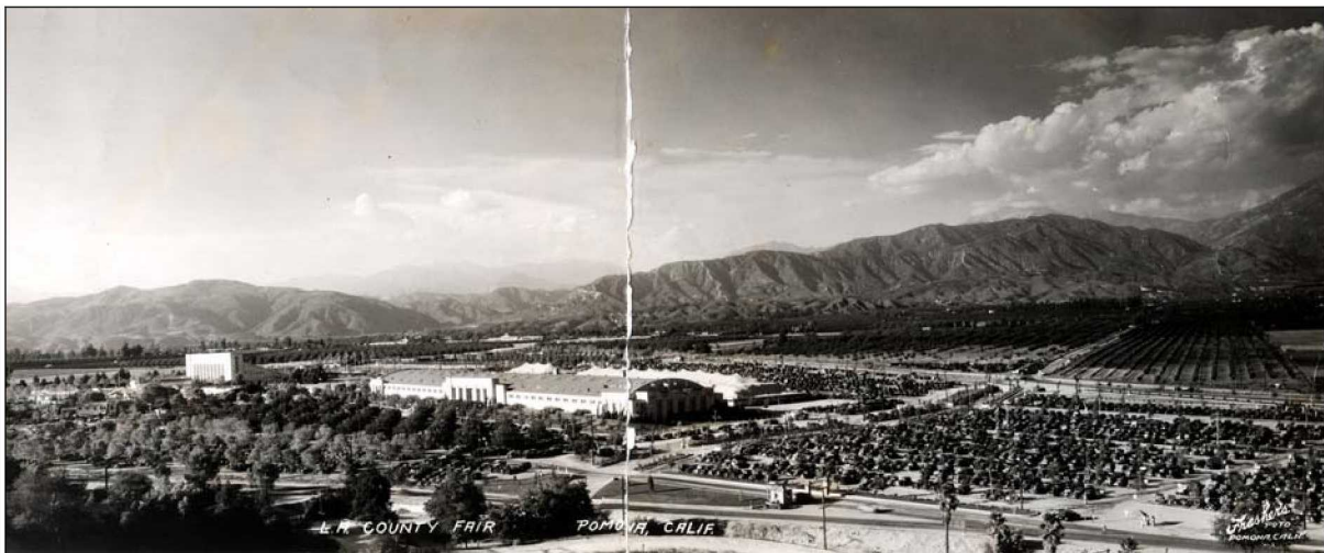
Figure 5: Exhibits Building 1932, with grandstand on the left side of the photograph (Source: Pomona Fairplex Archives).
