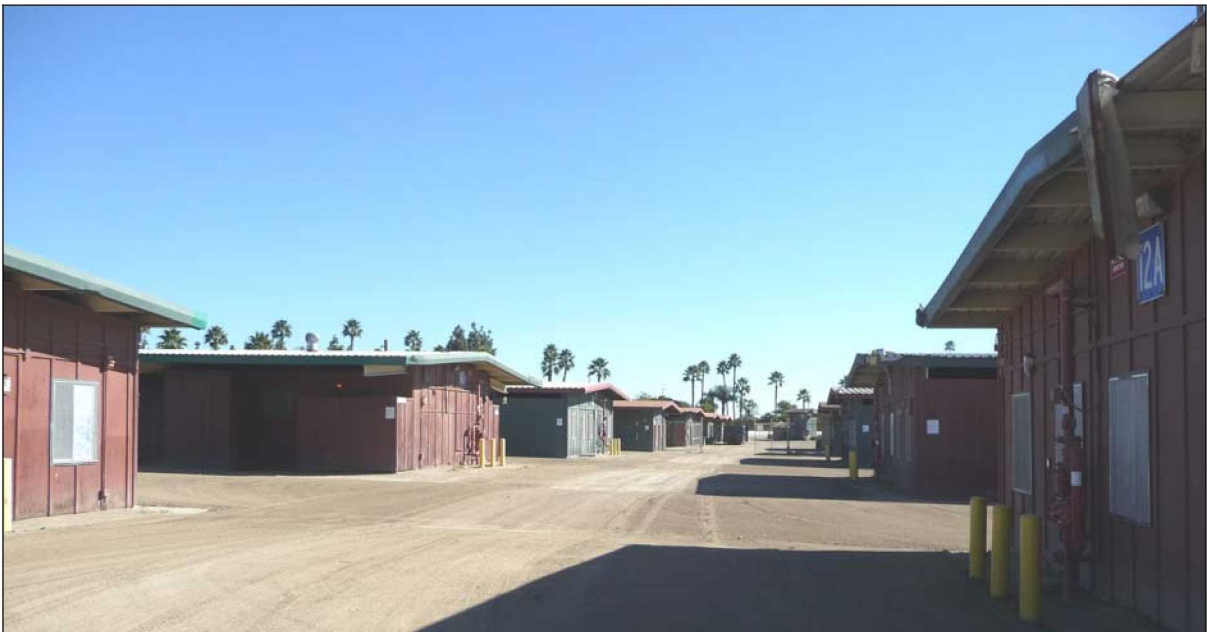
Figure 36: Horse Racing Stables central corridor between HRS 1-12A, view to the east (1/21/2011).
