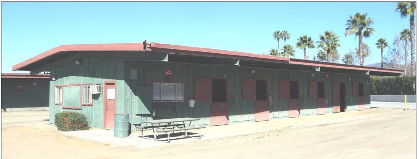
HRS #2 (also known as the office), view to the north (1/21/2011).
