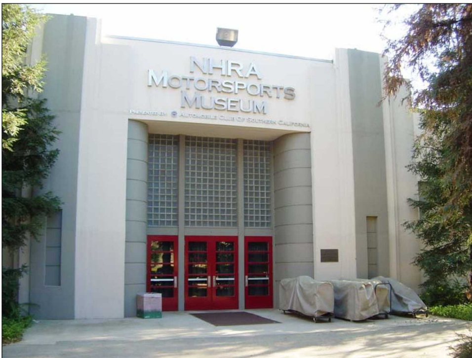
North elevation entrance (1/21/11)
