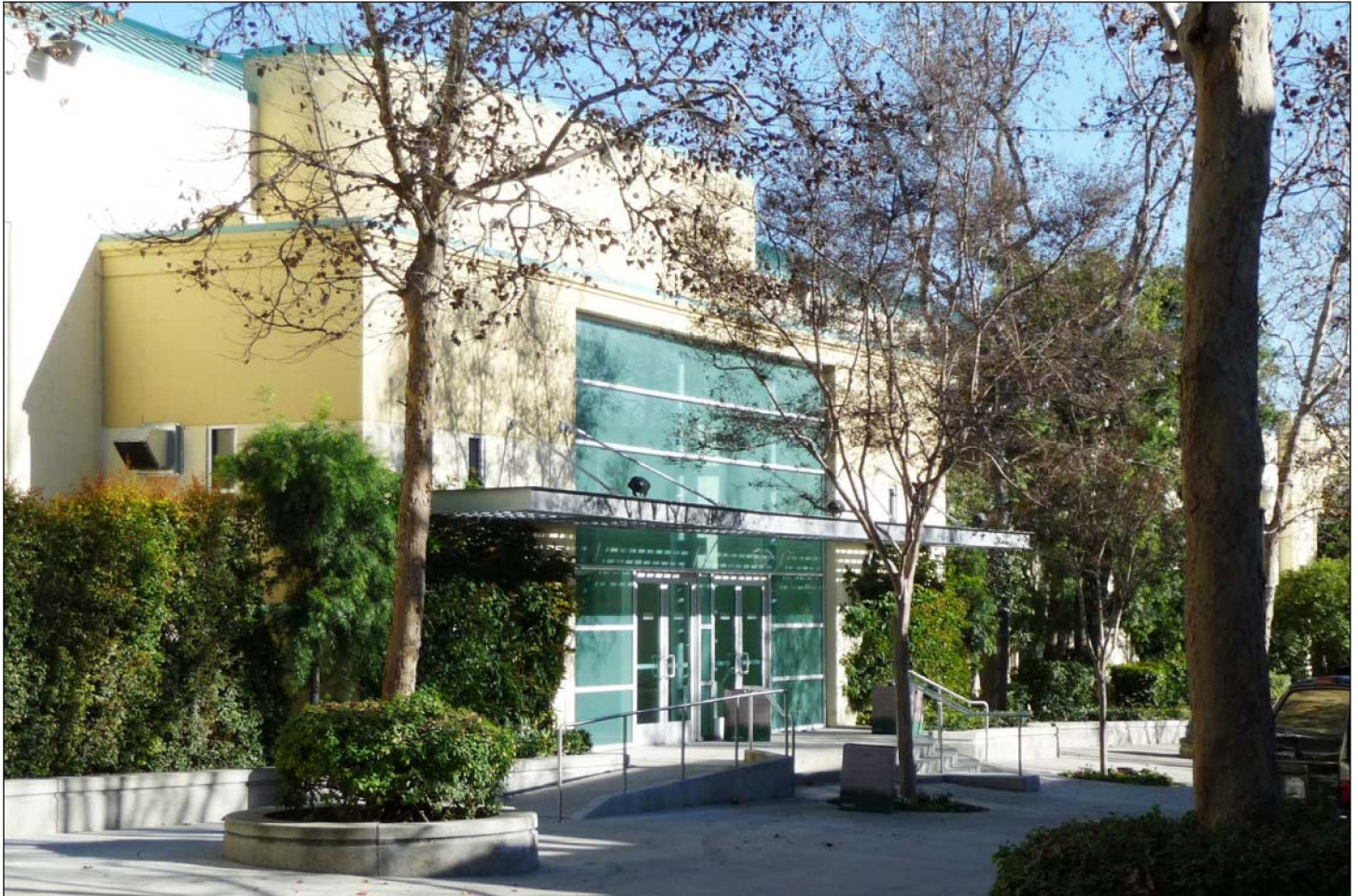
West elevation of Building #9 (1/21/11).
