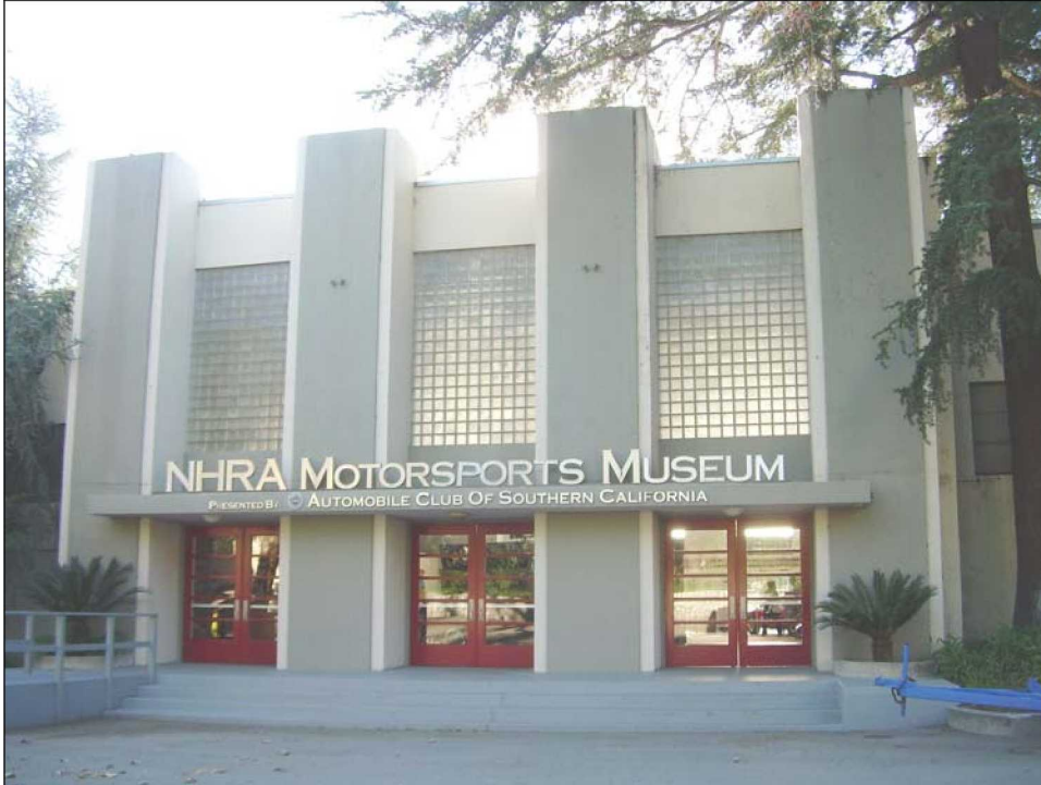
East elevation entrance (1/21/11)
