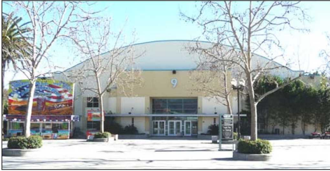
Figure 42: Barrel-Roofed Building #9, north elevation (1/21/11).
