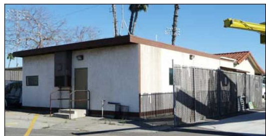
Figure 45: Security Office addition, view to the southeast (1/21/11).
