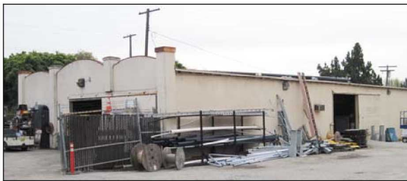
Figure 49: Facilities Yard building, view to the southeast (3/2/11).
