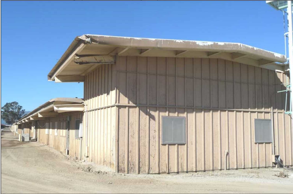
View to the north (1/21/11).
