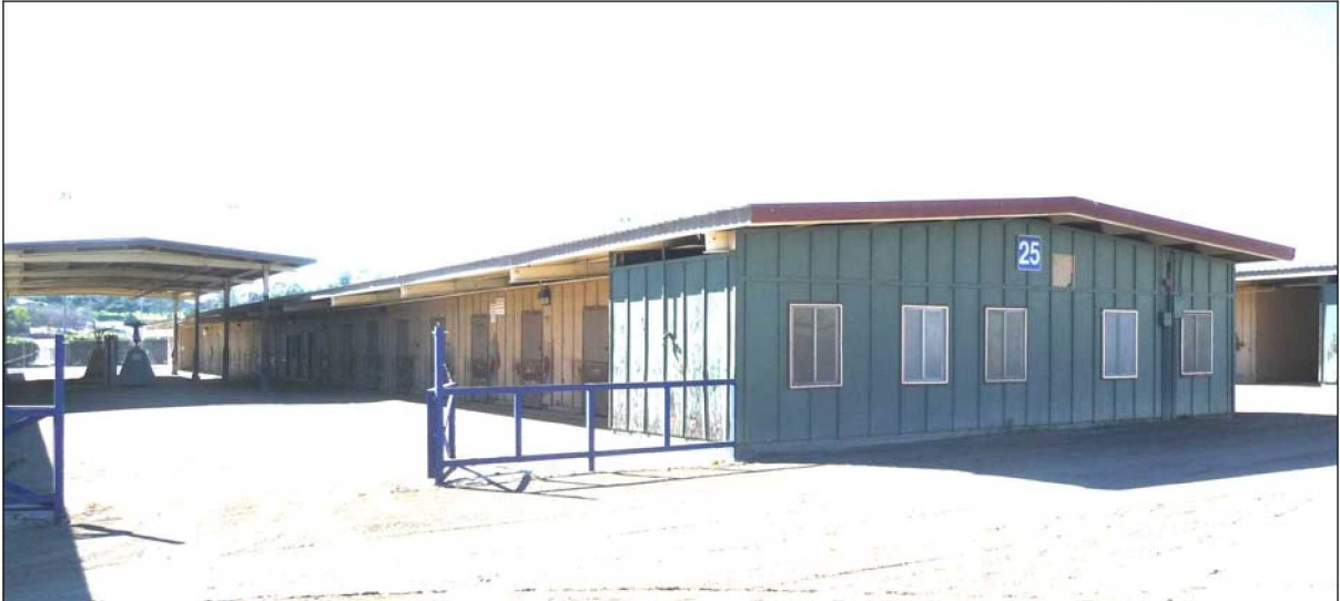
Figure 37: Horse Racing Stable #25, view to the west; note metal canopy between stables (1/21/2011). This building is representative of HRS 14–28.
