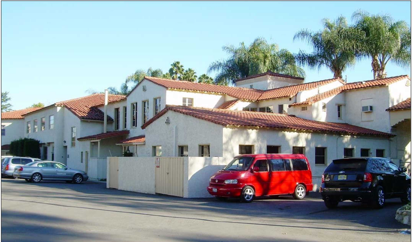
North elevation, view to the southeast (1/21/11)
