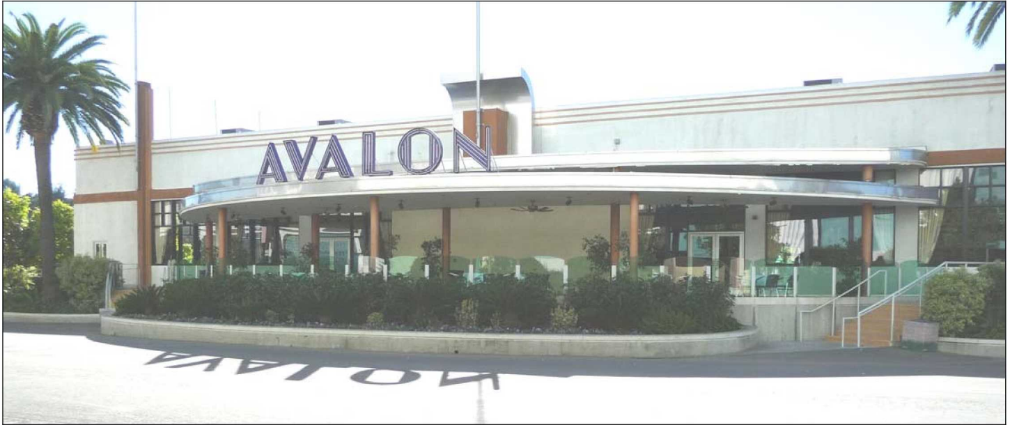
East elevation with modern Art Deco patio cover (1/21/11)
