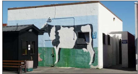
Figure 54: Free-standing restroom in the livestock area, view to the northeast (1/21/11).
