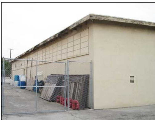
Building 4, view to the north (3/2/11).
