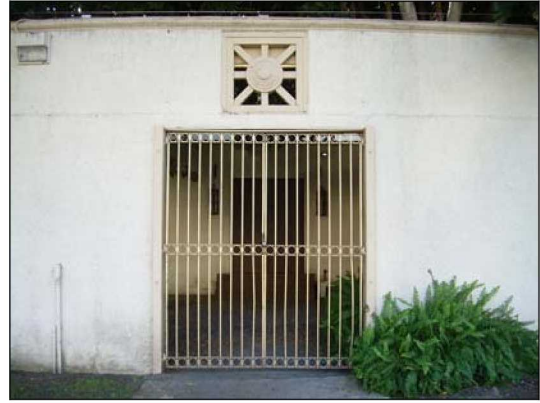
Figure 22: Millard Sheets Building wall detail, east elevation (1/21/11).
