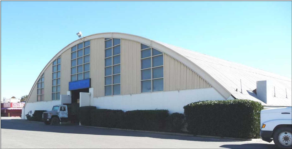
Figure 58: Quonset Hut #10, view to the southeast (1/21/11).
