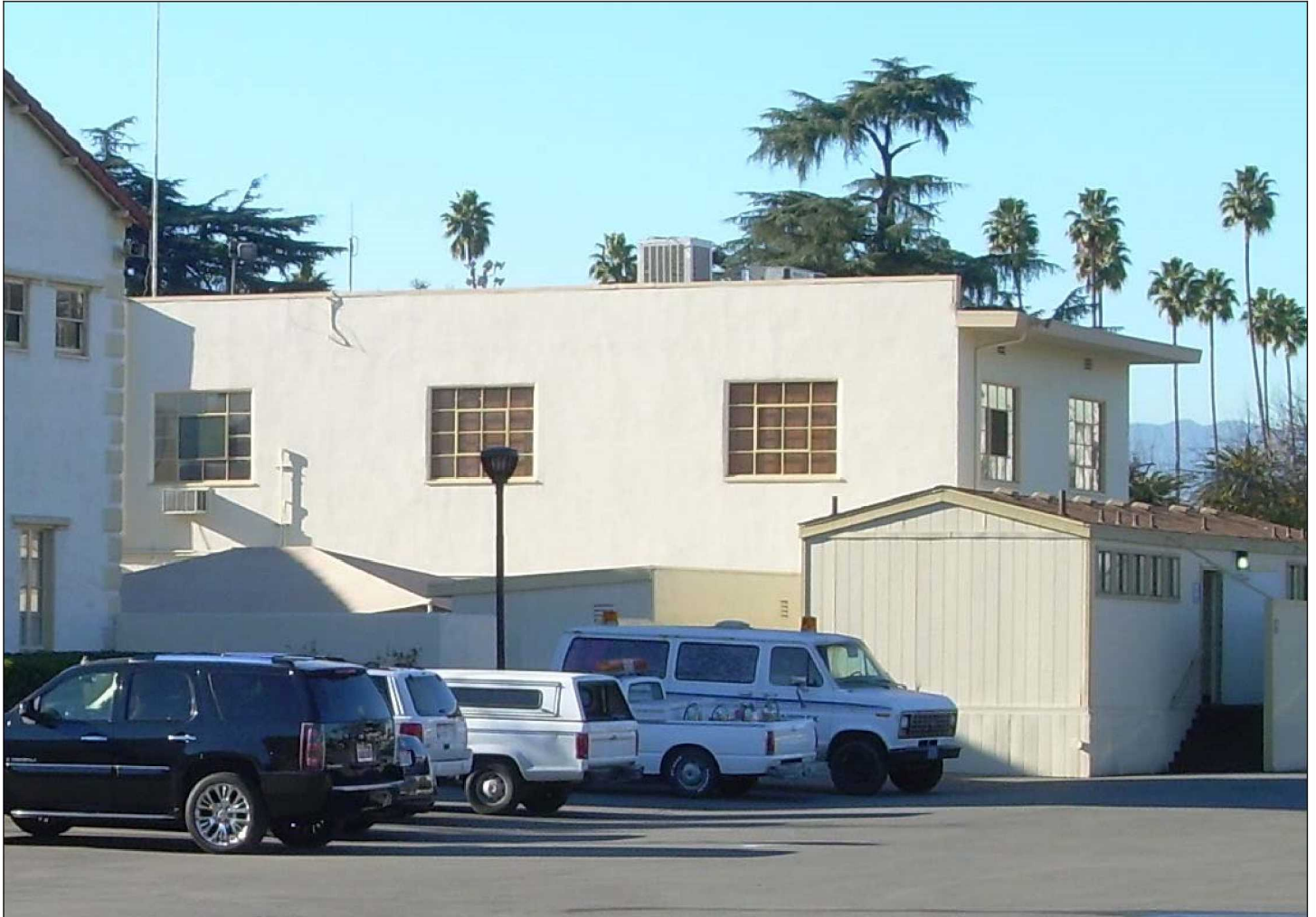
South elevation (1/21/11). Part of the Administration Building 2 is in the foreground (left side of photograph).
