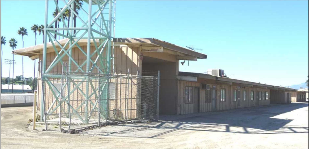
Figure 60: Race Official's Office, view to the northwest (1/21/11).
