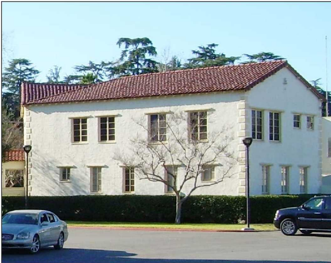
Figure 18: Administration Building 2, south and east elevations (1/21/11).
