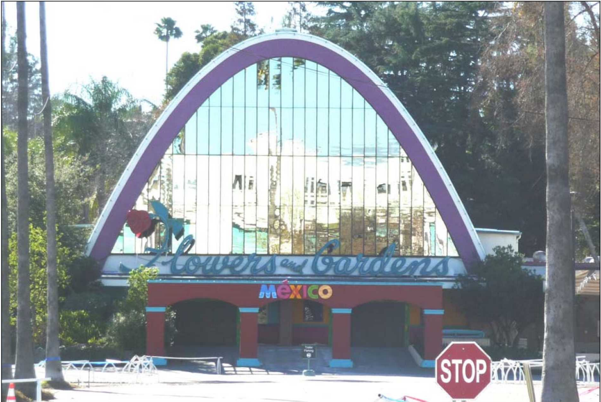
Figure 39: Flower Building, view to the southwest (1/21/11).
