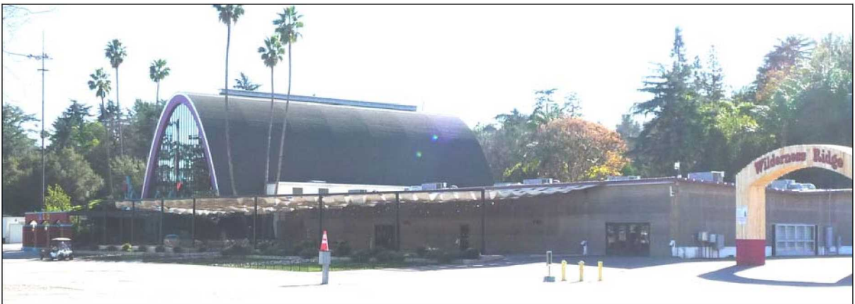
Figure 40: Flower Building, view to the south (1/21/11).
