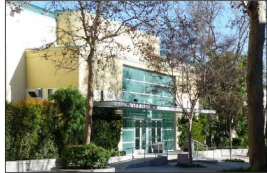
Figure 43: Barrel-Roofed Building #9, west elevation (1/21/11).
