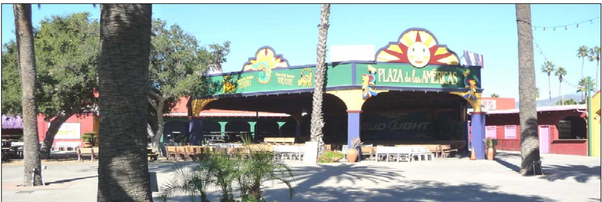
Figure 55: Plaza de las Americas, view to the north (1/21/11).
