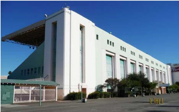
Figure 15: Grandstand, western elevation, view to the southeast (1/21/11).
