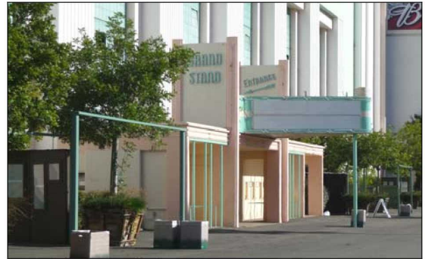
Figure 16: Grandstand main entrance, view to the southeast (1/21/11).
