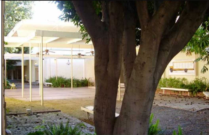
Courtyard area on east side of building, view to the south (1/21/11)
