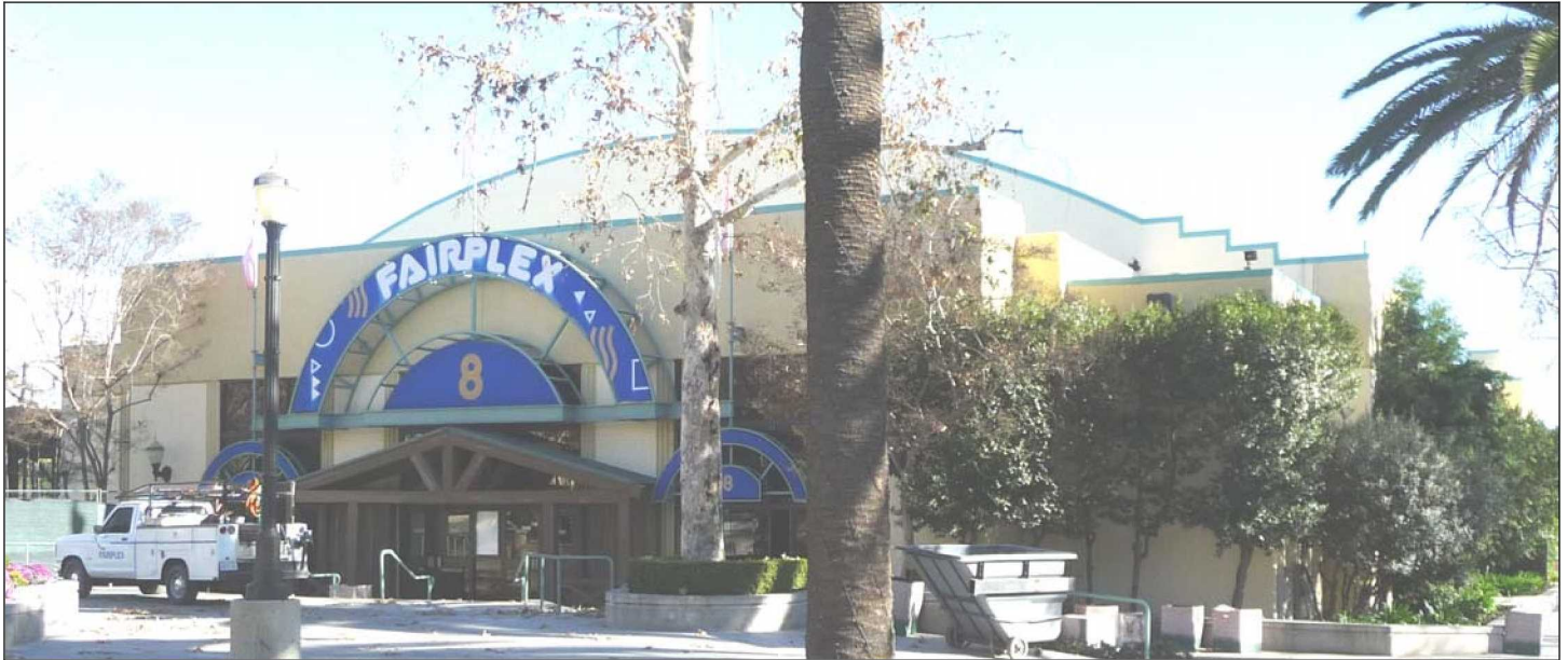
Northwest elevation of Building 8, which is slightly different from northwest elevations of Buildings 5-7 (1/21/11).
