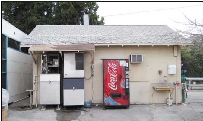
Building 2, view to the east (3/2/11).
