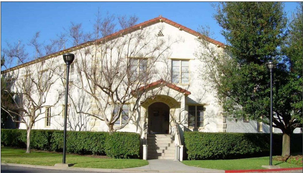
Figure 17: Administration Building 2, southwest elevation (1/21/11).
