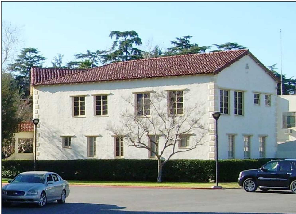
South and east elevations (1/21/11)
