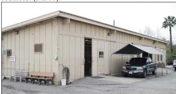
Figure 51: Facilities Yard building with board-and-batten siding, view to the south (3/2/11).
