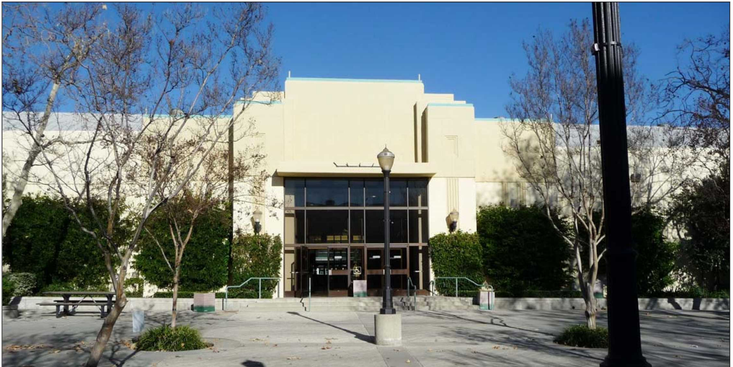
West elevation entrance of Building 7. This is representative of most of the east and west elevation entrances on Buildings 5-8 (1/21/11).
