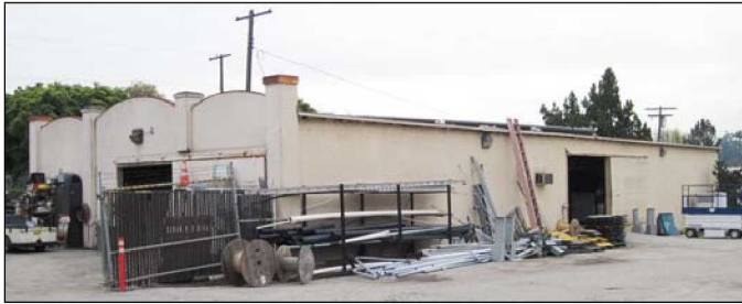
Building 1, view to the southeast (3/2/11).
