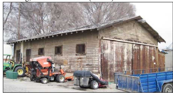
Figure 52: Facilities Yard wood-frame building, view to the northeast (3/2/11).
