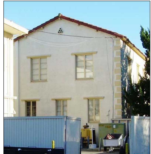
Figure 19: Administration Building 2, north elevation (1/21/11).
