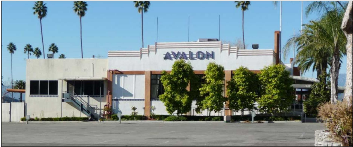
Figure 28: Avalon, south elevation showing pre-1948 addition (1/21/11).
