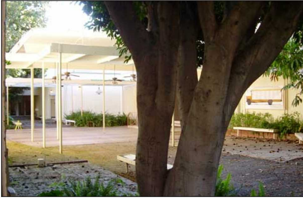
Figure 21: Millard Sheets Building courtyard, east side of building, view to the south (1/21/11).
