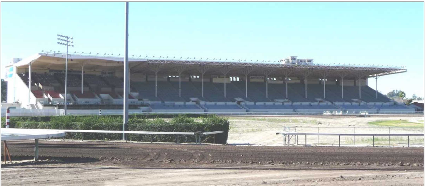
Trackside view of grandstand, view to the west (1/21/2011)
