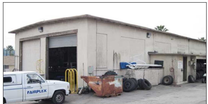
Building 7, view to the south (3/2/11).
