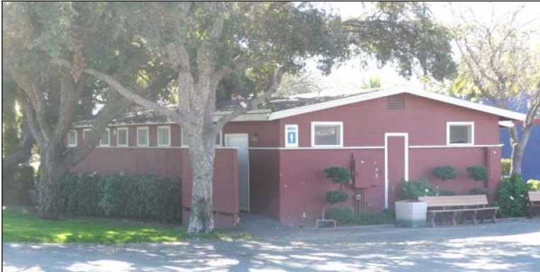
Restroom adjacent to White Avenue, northeast of Plaza de las Americas (1/21/2011).
