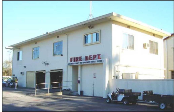
Figure 48: Fire Station, view to the southeast (1/21/11).
