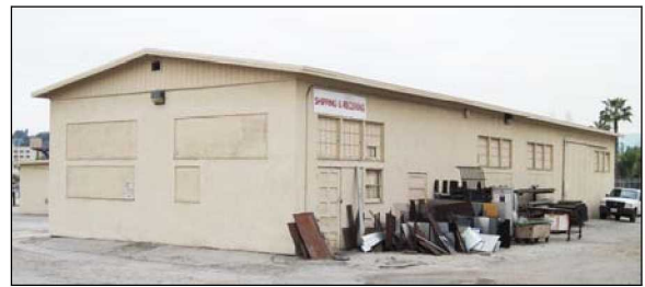
Figure 50: Facilities Yard shipping and receiving building, view to the south (3/2/11).
