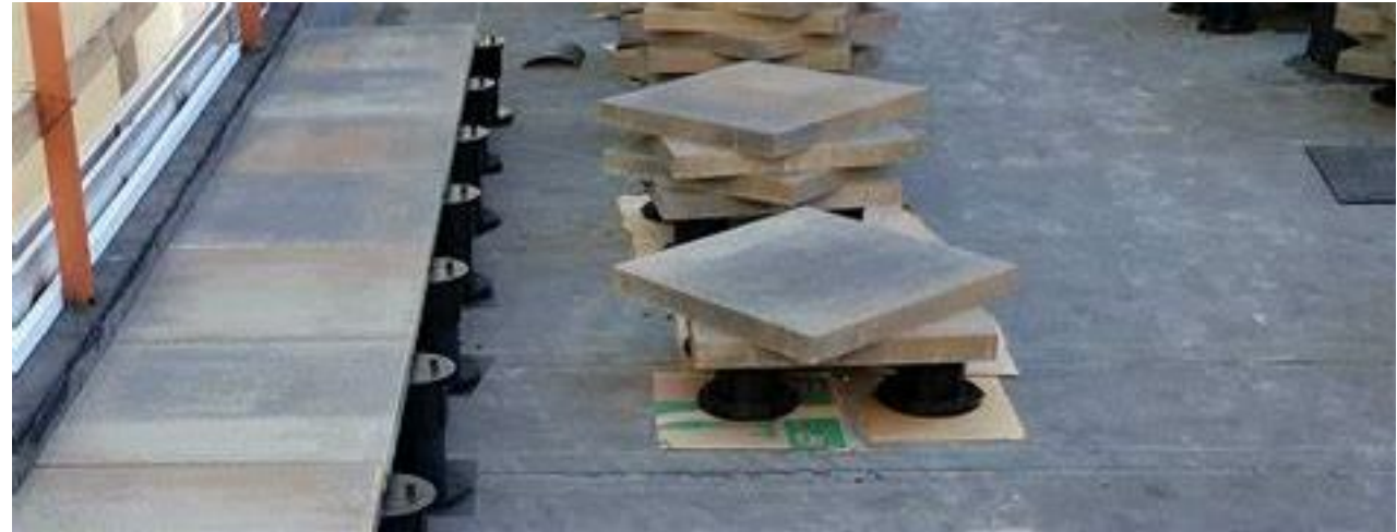
8 ORCO DECK ON PEDESTALS OVER ROOF
