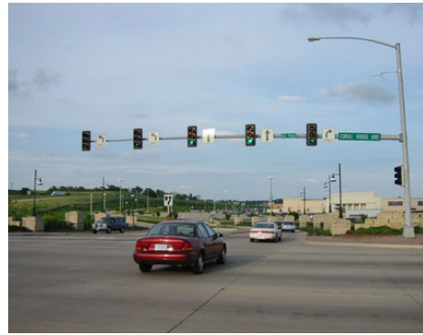
CONVERT SIGNAL TO MAST ARM (FROM PEDESTAL-MOUNTED)
