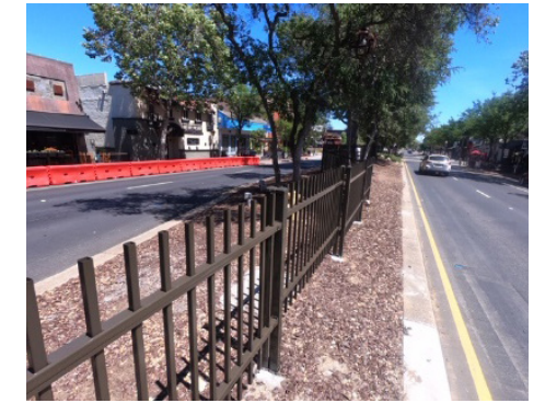
INSTALL PEDESTRIAN MEDIAN FENCING ON APPROACHES
