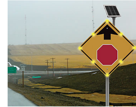
INSTALL FLASHING BEACONS AS ADVANCE WARNING
