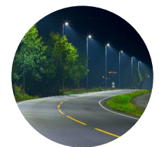
Upgrade Street Lighting (install new street light poles) Enhance Nighttime Visibility & Safety
