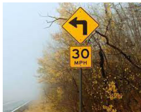
INSTALL CURVE ADVANCE WARNING SIGNS
