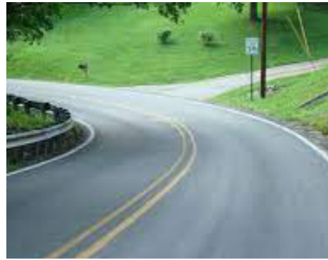
IMPROVE HORIZONTAL ALIGNMENT (FLATTEN CURVES)
