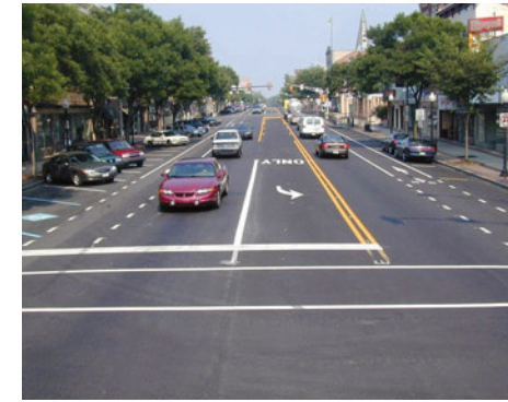
ROAD DIET (REDUCE TRAVEL LANES AND ADD A TWO WAY LEFT-TURN AND BIKE LANES)
