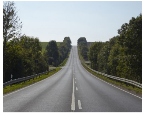
FLATTEN CREST VERTICAL CURVE
