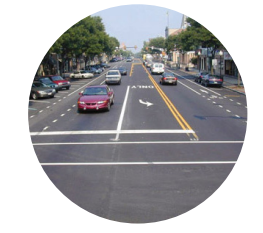
Install Pavement Marking Enhance Arrow & Pavement Legend Visibility
