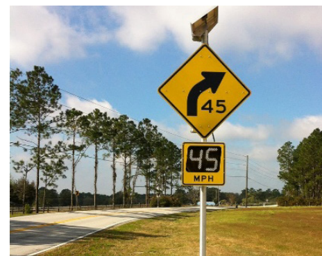
INSTALL DYNAMIC/VARIABLE SPEED WARNING SIGNS
