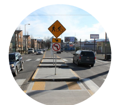
New Signage & Striping Enhance Sign & Striping Visibility for Added Safety
