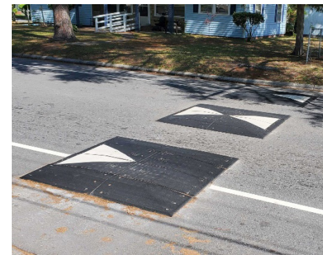
SPEED CUSHIONS, SPEED HUMPS AND SPEED TABLES
