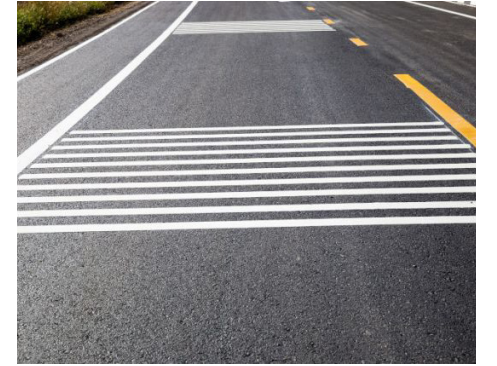
INSTALL TRANSVERSE RUMBLE STRIPS ON APPROACHES
