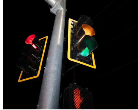
IMPROVE SIGNAL HARDWARE: LENSES, BACK-PLATES WITH RETROREFLECTIVE BORDERS, MOUNTING, SIZE, AND NUMBER
