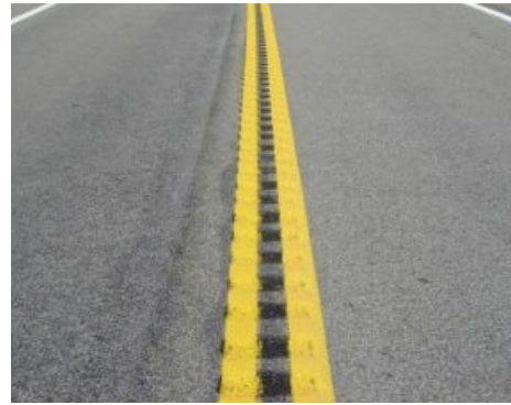
INSTALL CENTERLINE RUMBLE STRIPS/STRIPES
