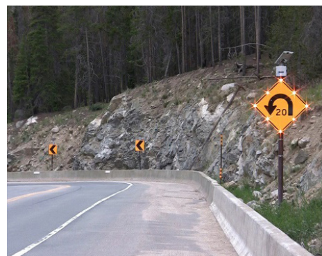
INSTALL CURVE ADVANCE WARNING SIGNS (FLASHING BEACON)
