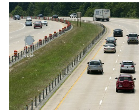
INSTALL MEDIAN BARRIER
