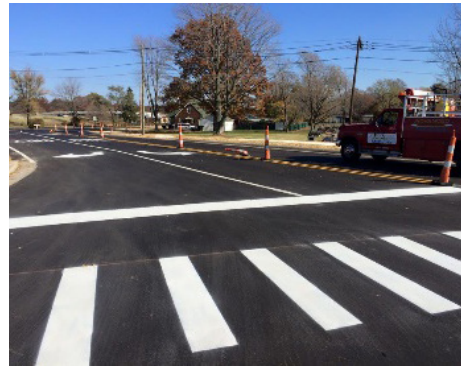
INSTALL ADVANCE STOP BAR BEFORE CROSSWALK
