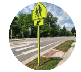
New Sign Post Ensure Proper Sign Placement & Fix Knocked over Signs
