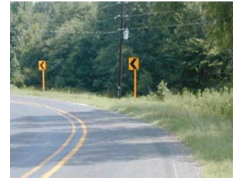
INSTALL CHEVRON SIGNS ON HORIZONTAL CURVES
