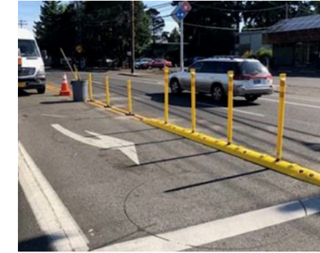
INSTALL LEFT-TURN LANE AND/OR ADD TURN PHASE (SIGNAL HAS NO LEFT-TURN LANE OR PHASE BEFORE)
