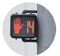
New Countdown Pedestrian Signal Head / Push Buttons Enhances Pedestrian Safety
