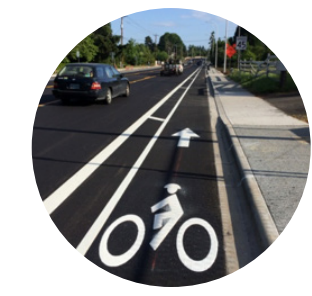
Install Class II Buffered Bike Lane Enhance Bicyclist Safety / Comfort & Separation from Traffic
