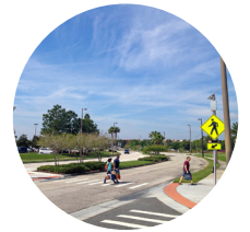
Improve Pedestrian Crossing with Bulbouts & ADA Curb Ramps Enhance Pedestrian Safety & Accessibility
