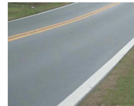
INSTALL EDGE LINES AND CENTERLINES
