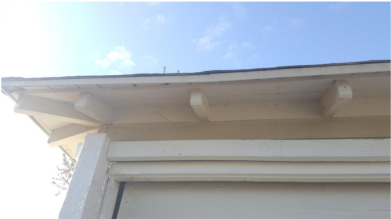
Rafters underneath the eaves of garage roof
