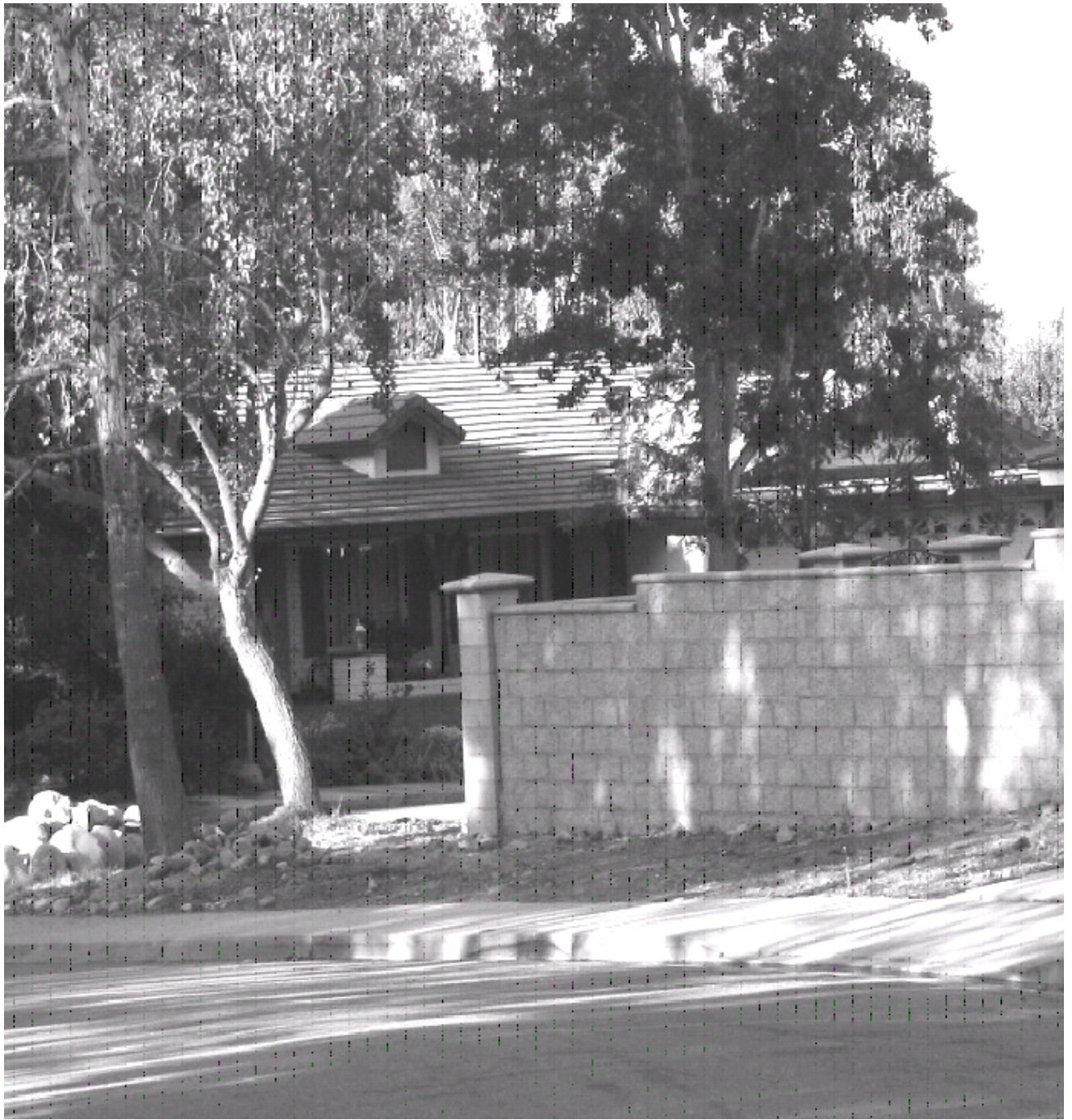
Split-faced decorative block wall with decorative cap along a street facing side property line
