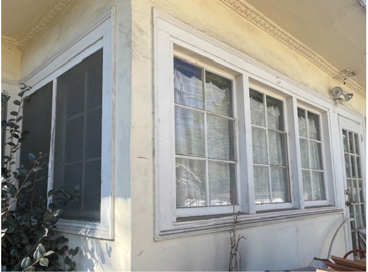
Existing kitchen windows
