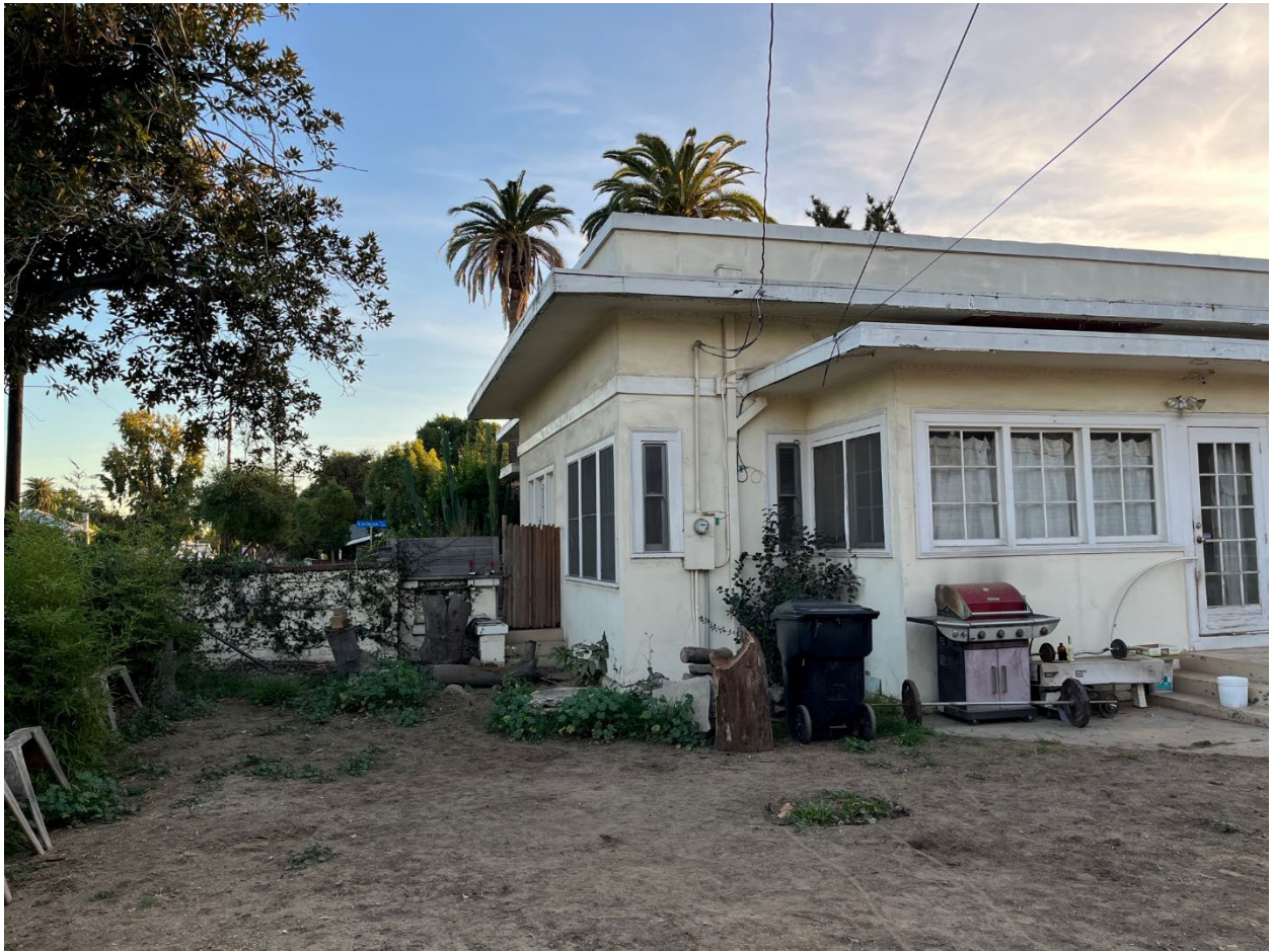
Rear of house showing the Existing Kitchen Windows
