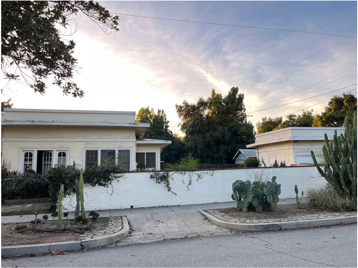
Street side of house showing the existing kitchen windows at rear of house
