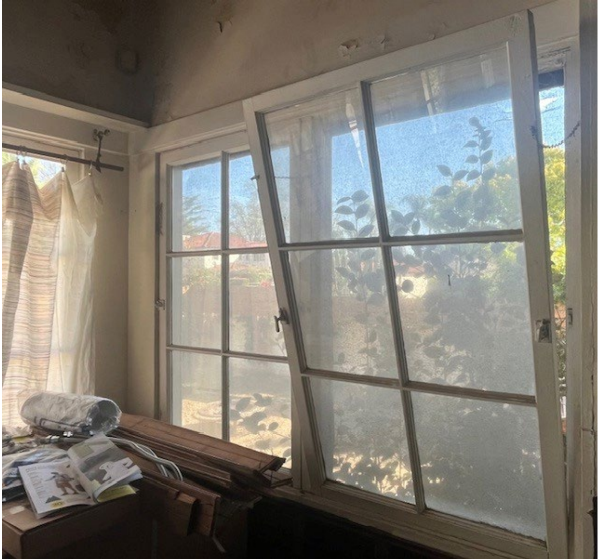
Existing kitchen windows
