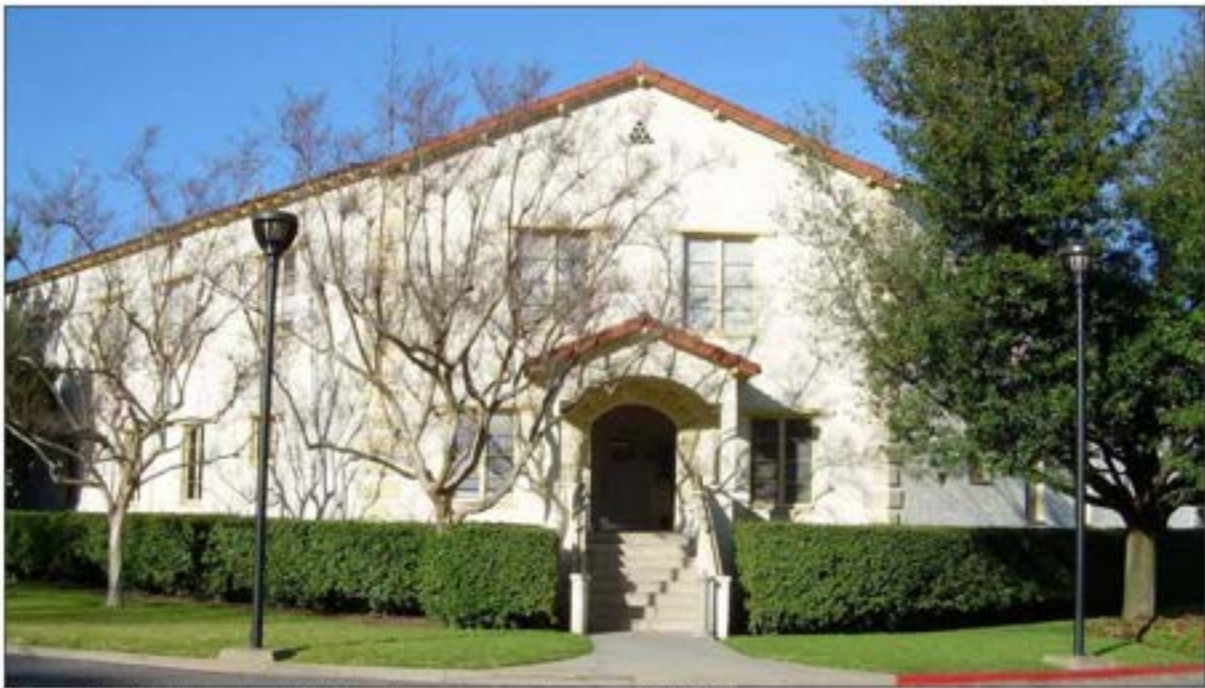
Figure 17: Administration Building 2, southwest elevation (1/21/11).
