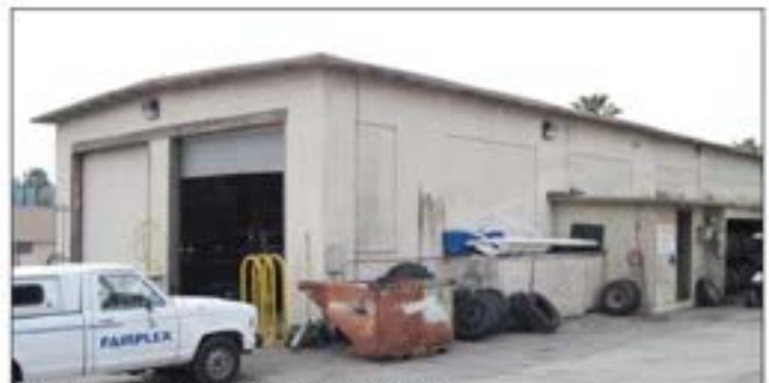
Building 7, view to the south (3/2/11).
