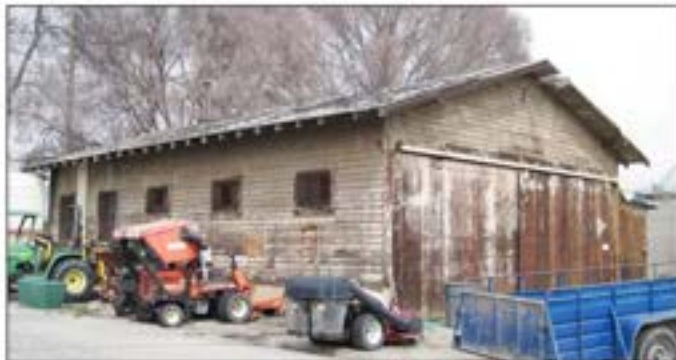
Building 8, view to the northeast (3/2/11).
