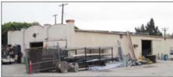
Figure 49: Facilities Yard building, view to the southeast (3/2/11).
