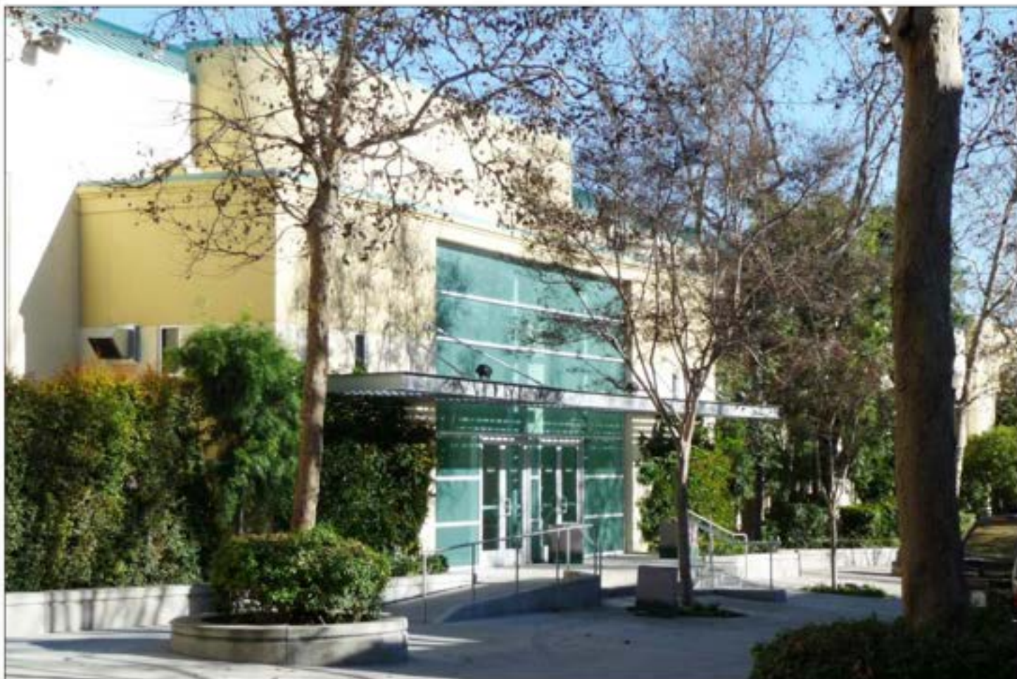
West elevation of Building #9 (1/21/11).
