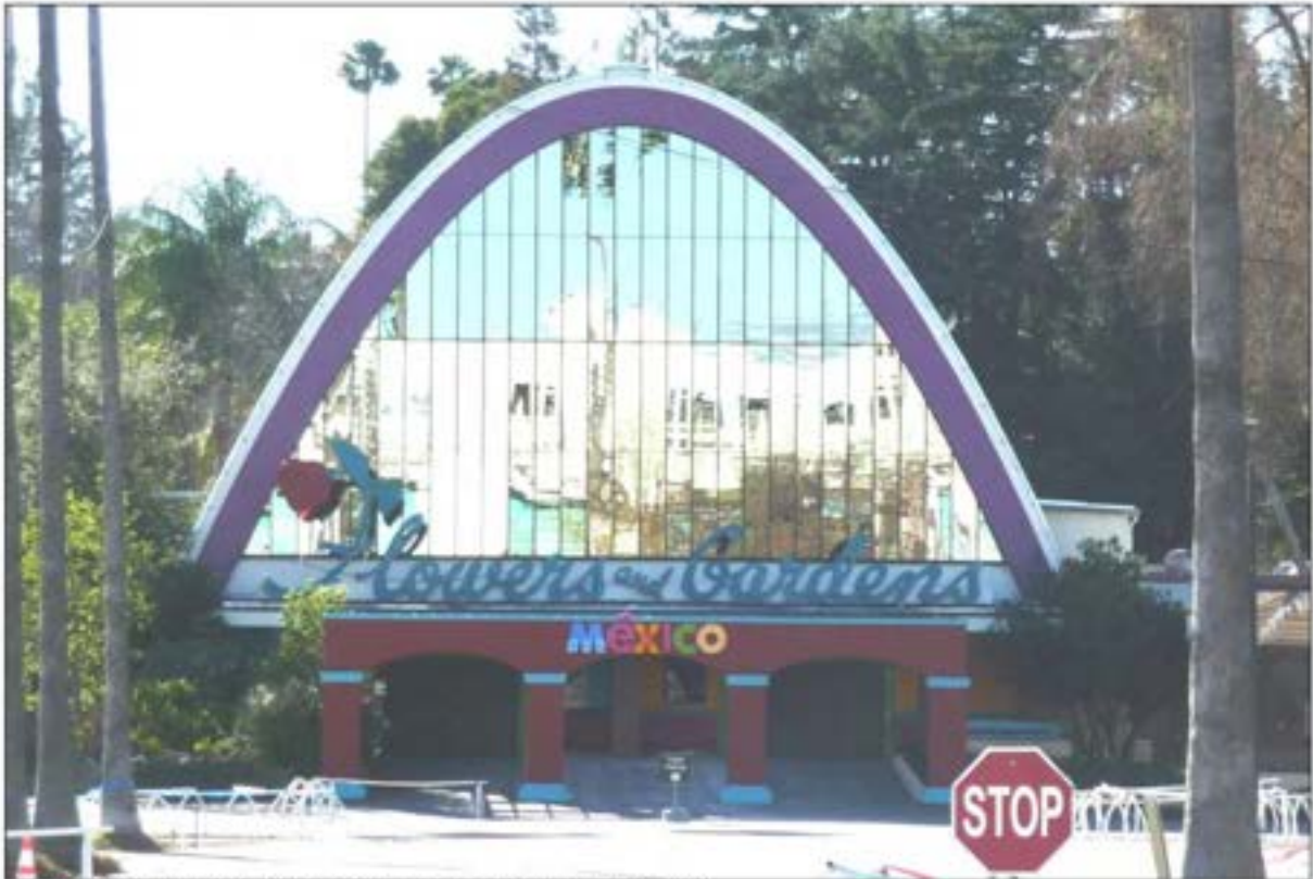
Figure 39: Flower Building, view to the southwest (1/21/11).
