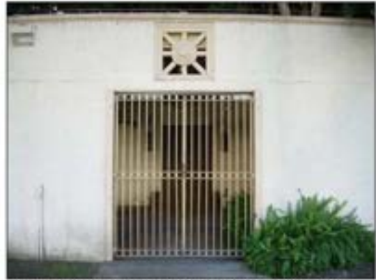
Figure 22: Millard Sheets Building wall detail, east elevation (1/21/11).
