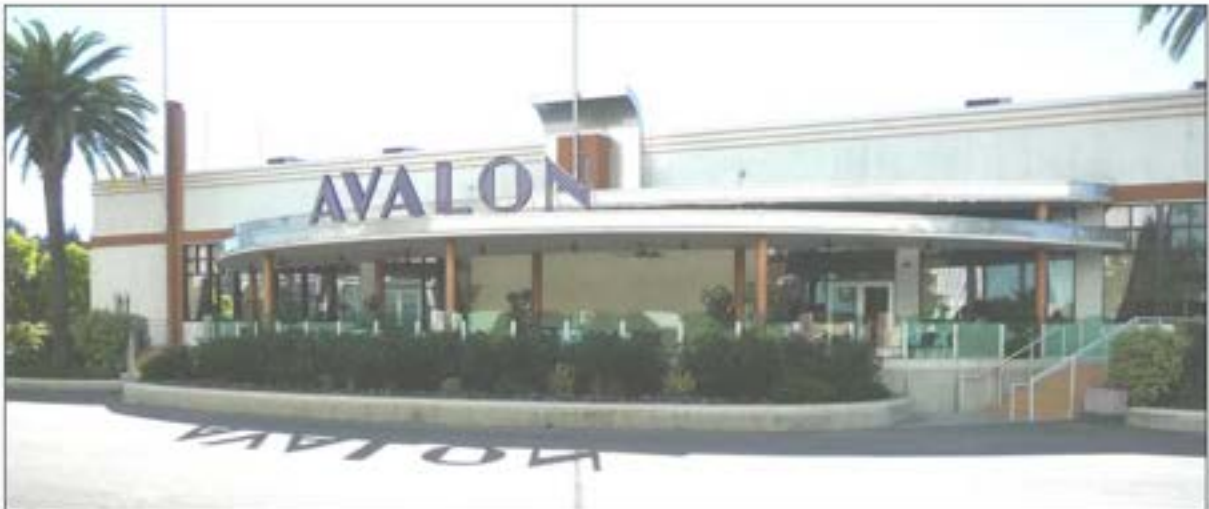
Figure 27: Avalon, east elevation with modern canopy/patio cover (1/21/11).
