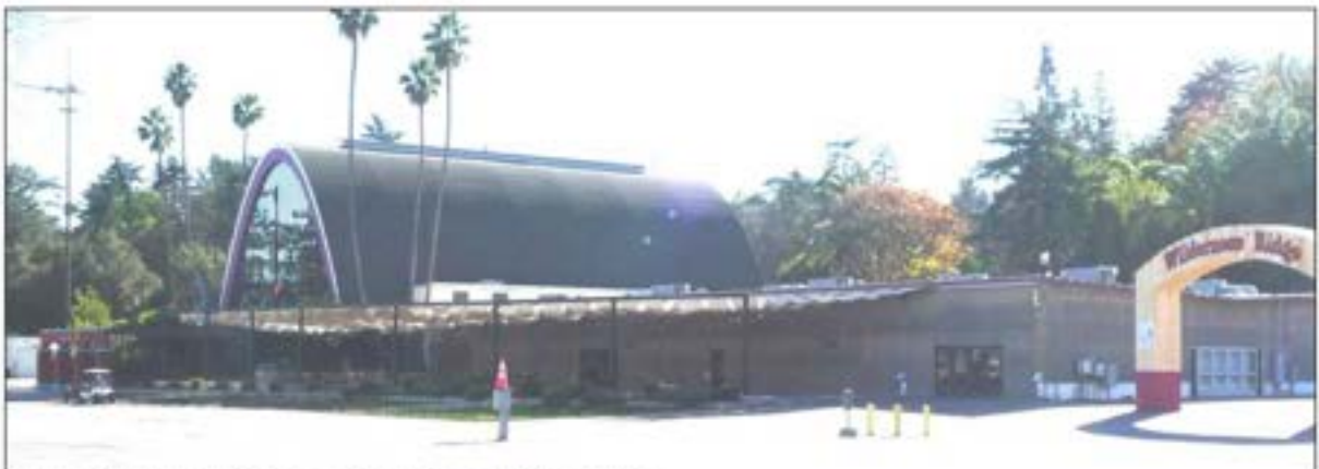
Figure 40: Flower Building, view to the south (1/21/11).
