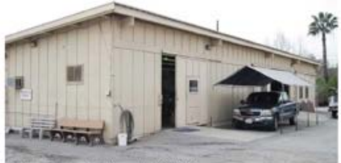
Building 5, view to the south (3/2/11)
