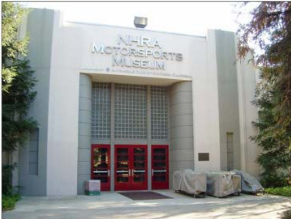
North elevation entrance (1/21/11)
