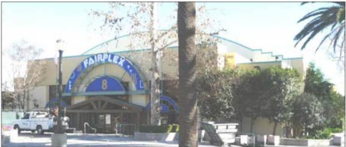
Figure 25: WPA barrel-roofed Exhibition Hall #8, northwest elevation (1/21/11).
