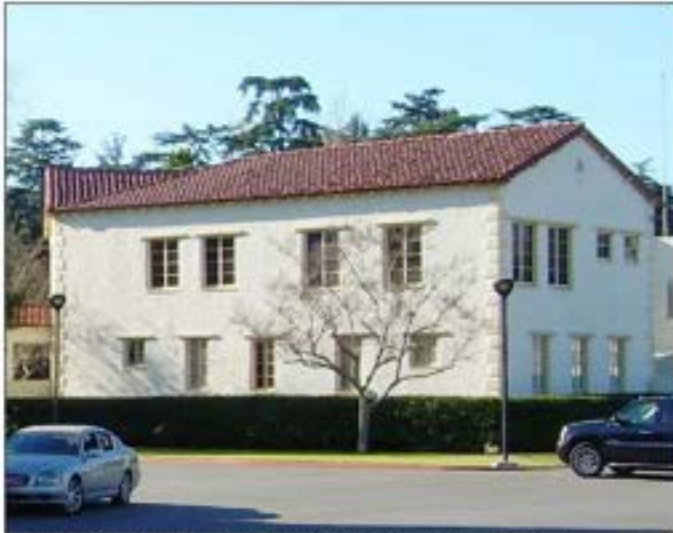
Figure 18: Administration Building 2, south and east elevations (1/21/11).
