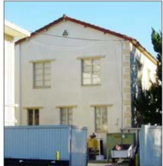
Figure 19: Administration Building 2, north elevation (1/21/11).
