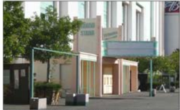
Figure 16: Grandstand main entrance, view to the southeast (1/21/11).
