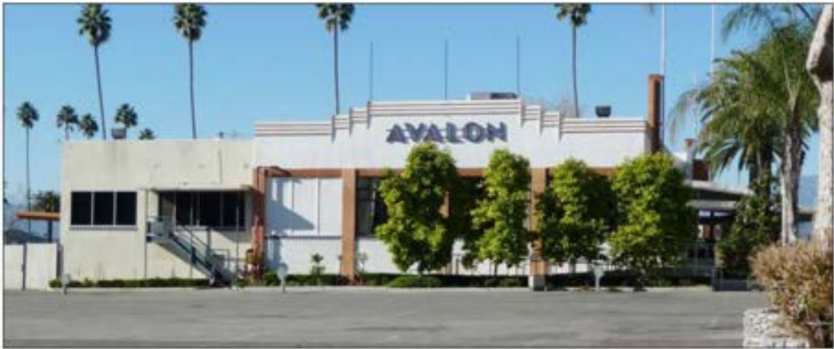
Figure 28: Avalon, south elevation showing pre-1948 addition (1/21/11).
