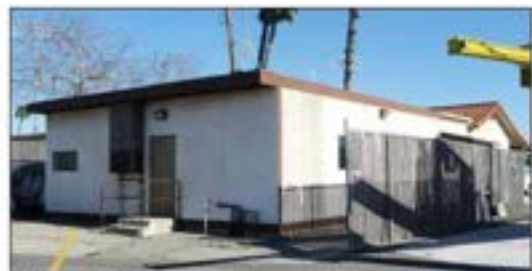
Figure 45: Security Office addition, view to the southeast (1/21/11).
