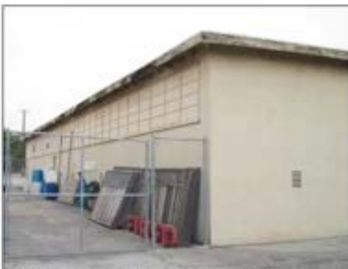
Building 4, view to the north (3/2/11).
