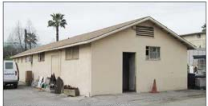
Building 6, view to the southwest (3/2/11).
