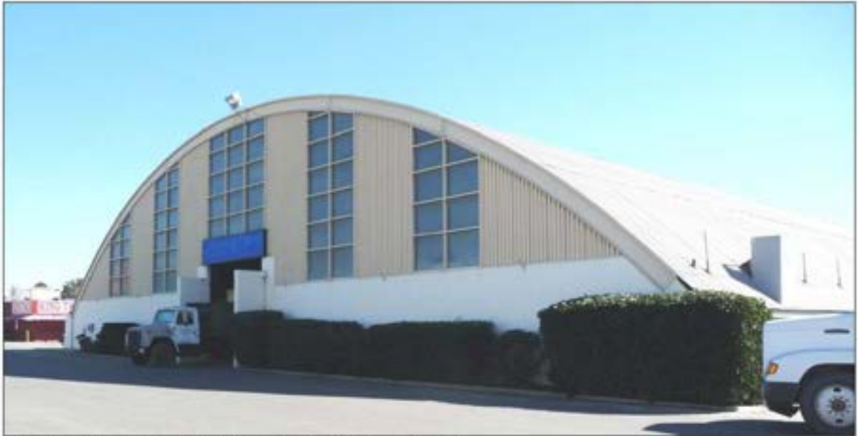
Figure 58: Quonset Hut #10, view to the southeast (1/21/11).
