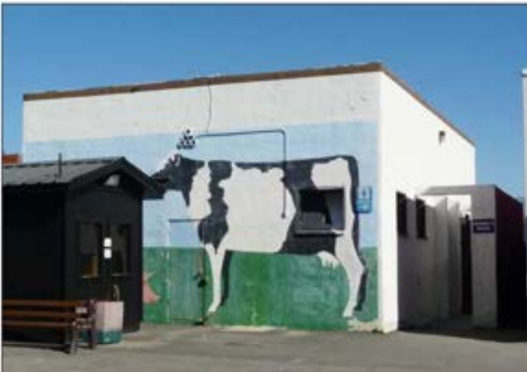
Restroom in the livestock area (1/21/11)
