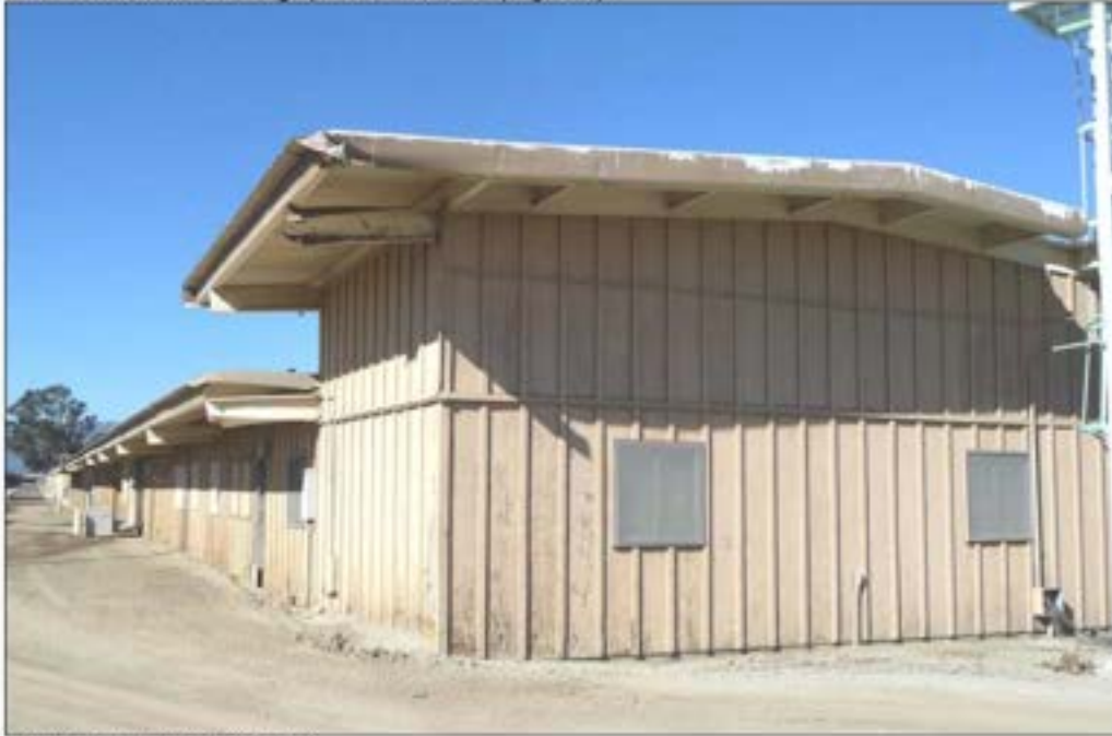
View to the north (1/21/11).
