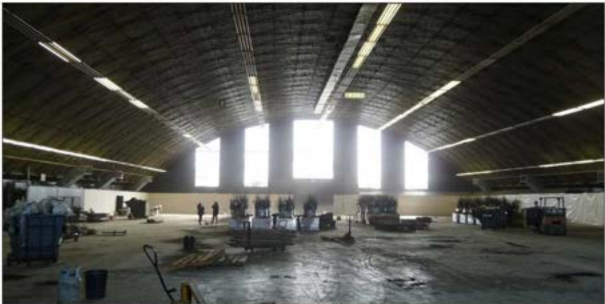
Figure 59: Quonset Hut #10 interior, view to the southeast (1/21/11).
