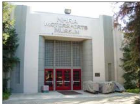
Figure 32: NHRA Motorsports Museum, north elevation entrance (1/21/11).
