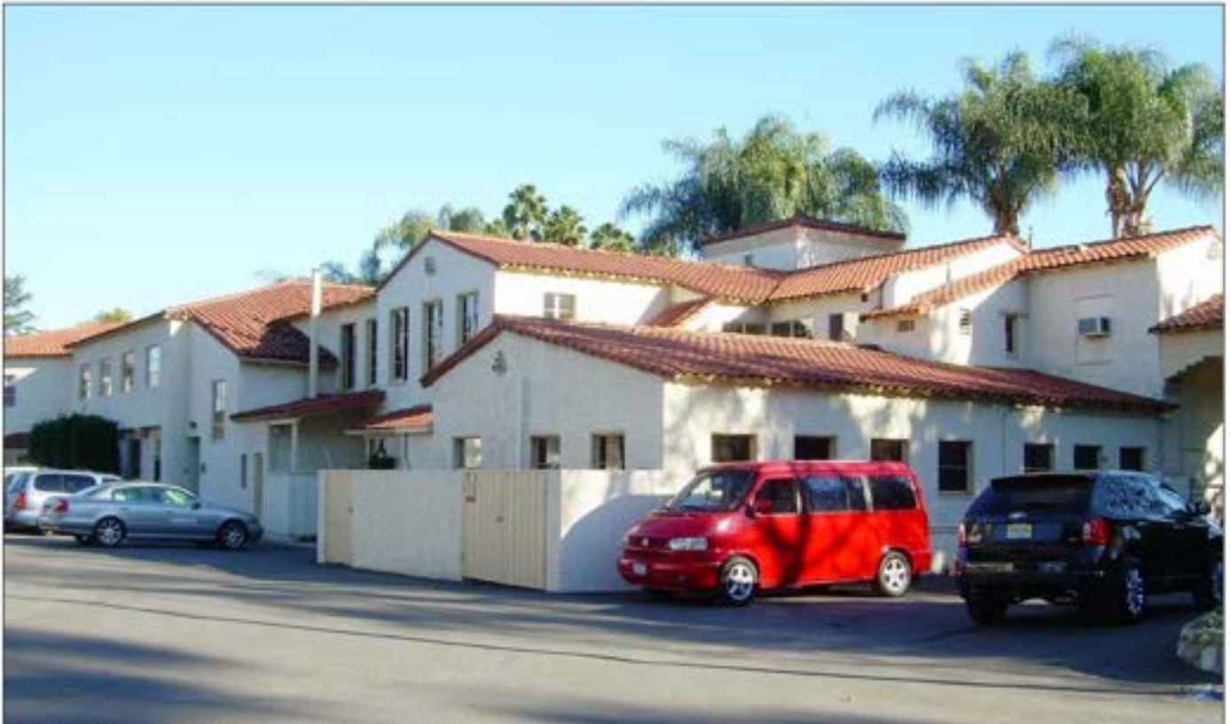
North elevation, view to the southeast (1/21/11)
