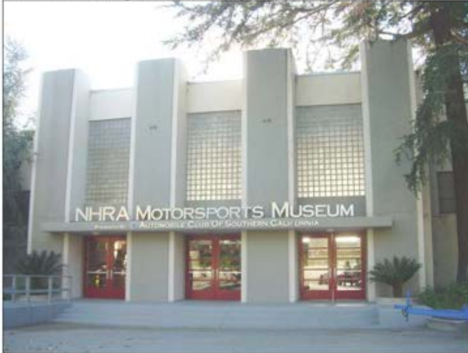
East elevation entrance (1/21/11)
