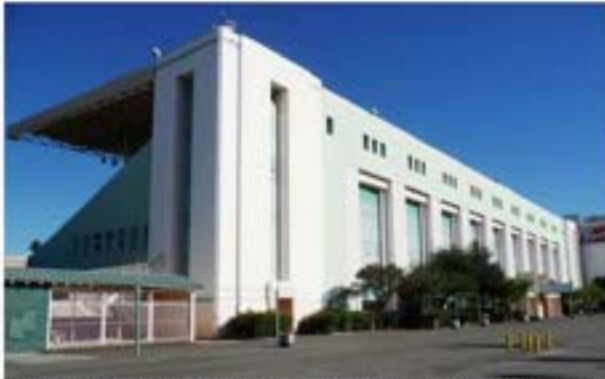
Figure 15: Grandstand, western elevation, view to the southeast (1/21/11).
