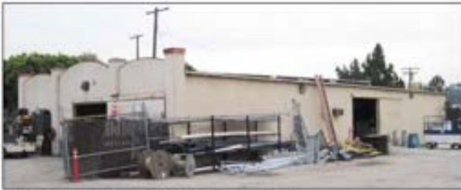
Building 1, view to the southeast (3/2/11).
