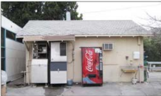
Building 2, view to the east (3/2/11).
