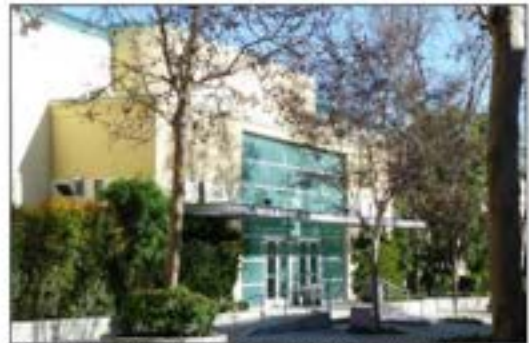
Figure 43: Barrel-Roofed Building #9, west elevation (1/21/11).
