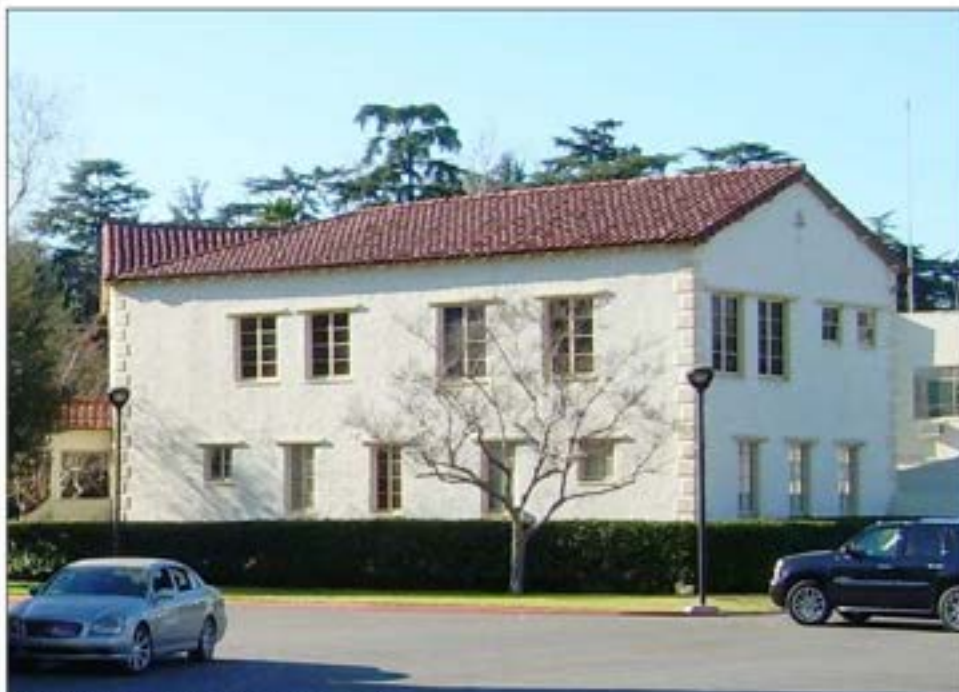
South and east elevations (1/21/11)
