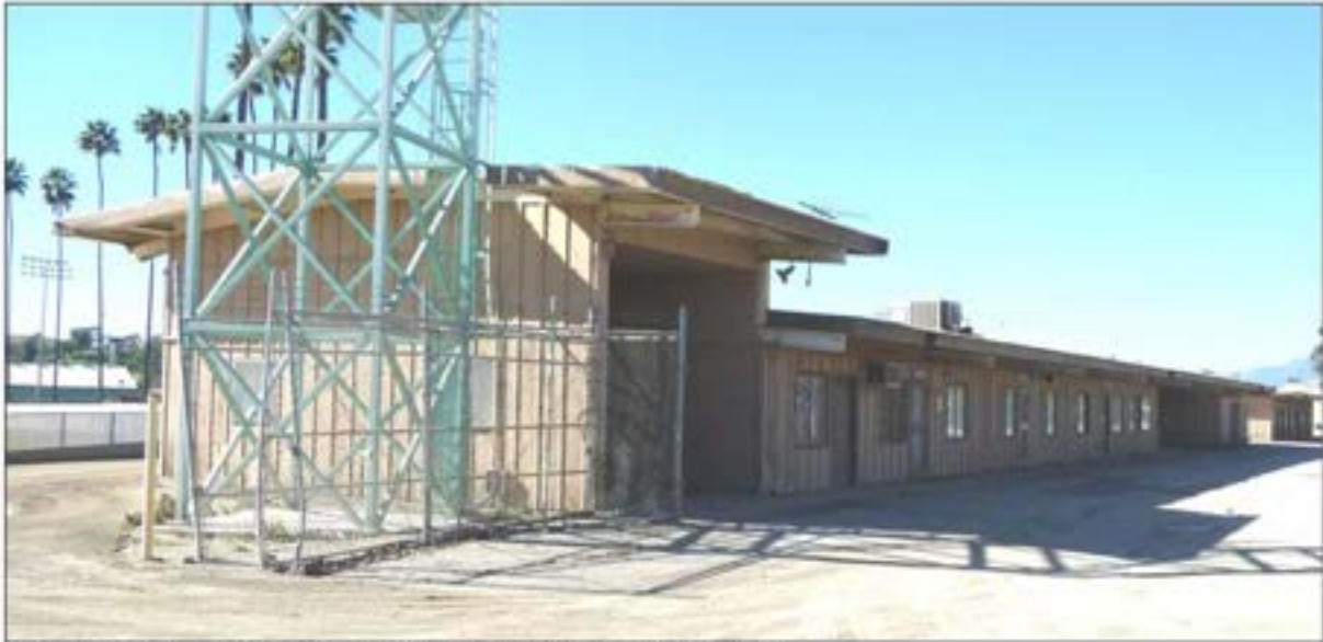
Figure 60: Race Official's Office, view to the northwest (1/21/11).
