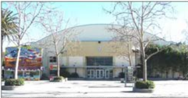
Figure 42: Barrel-Roofed Building #9, north elevation (1/21/11).
