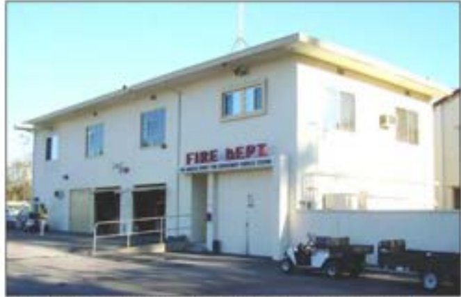
Figure 48: Fire Station, view to the southeast (1/21/11).
