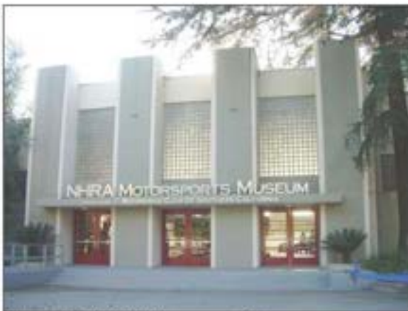
Figure 31: NHRA Motorsports Museum, east elevation entrance (1/21/11).
