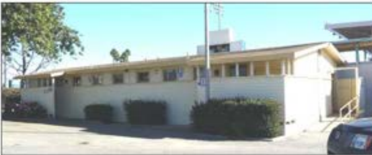
Restroom southeast of the security building (1/21/2011).
