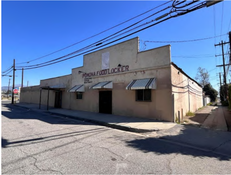
Exhibit 45. Example of a Commercial Building, 240 Oak Avenue
