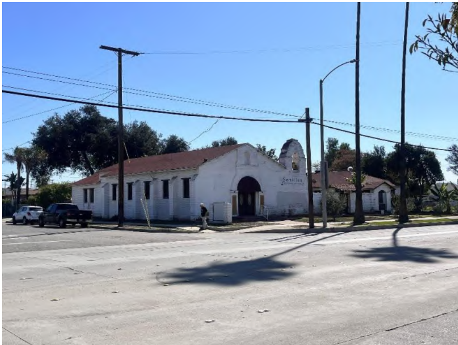
Exhibit 48. Mexican Congregational Church, 810 South White Street, constructed 1928
