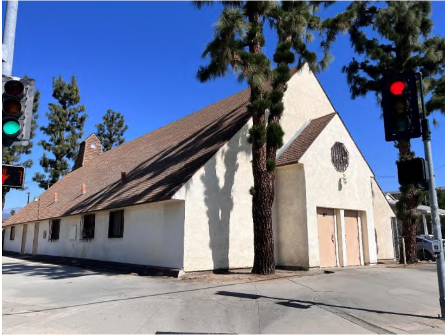
Exhibit 47. Sacred Heart Church, 1095 West Grand Ave, constructed 1935
