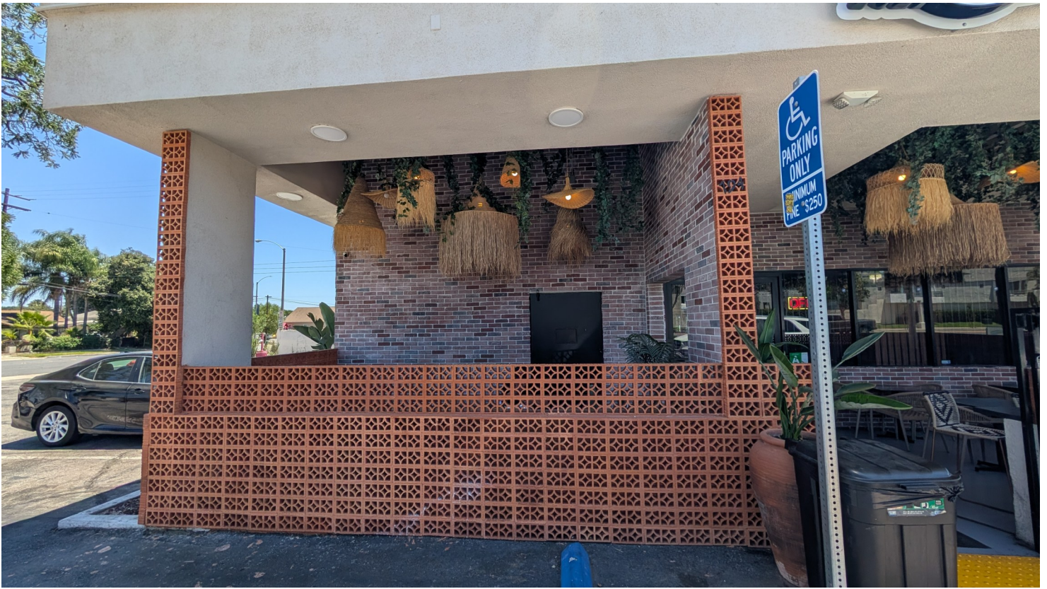
Description: Front façade of outdoor patio (east side) north elevation, facing E. Mission Blvd.
