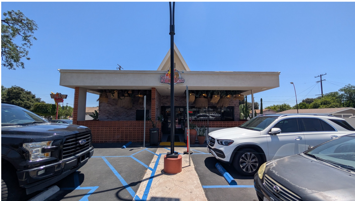
Description: Front façade, facing E. Mission Blvd.
